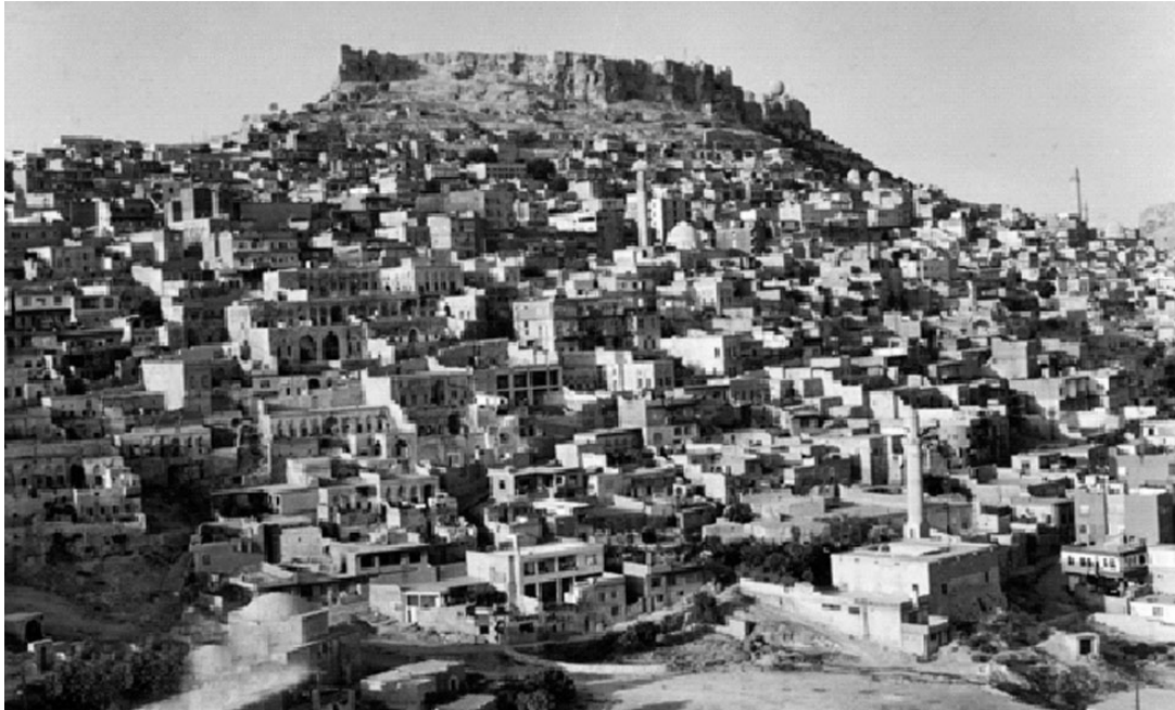
Fig 2.1 View of Mardin from the south (photograph: Adnan Avuka).
