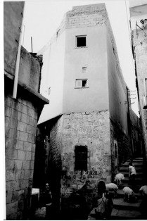
Fig. 5.8 The transition from masonry to plaster (photograph: Mert Kayasü).
