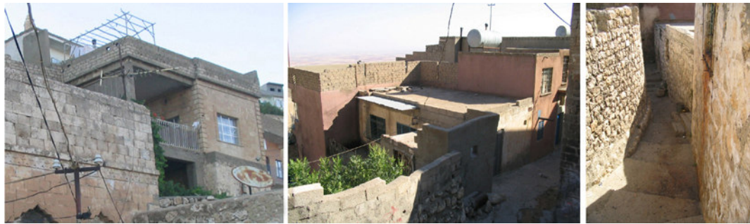
Fig. 5.1 The three buildings in parcels A, B and C respectively (photographs: Mert Kayasü).
