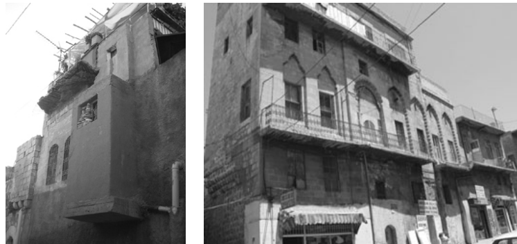
Fig. 4.18 The addition of a toilet to the main structure, elsewhere (photograph: Mert Kayasü).
