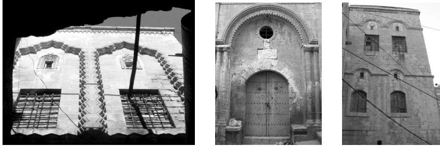
Fig. 4.9 The window and the top window ( kameriye ) embraced in the frame, Gözü House (photograph: Mert Kayasü).
