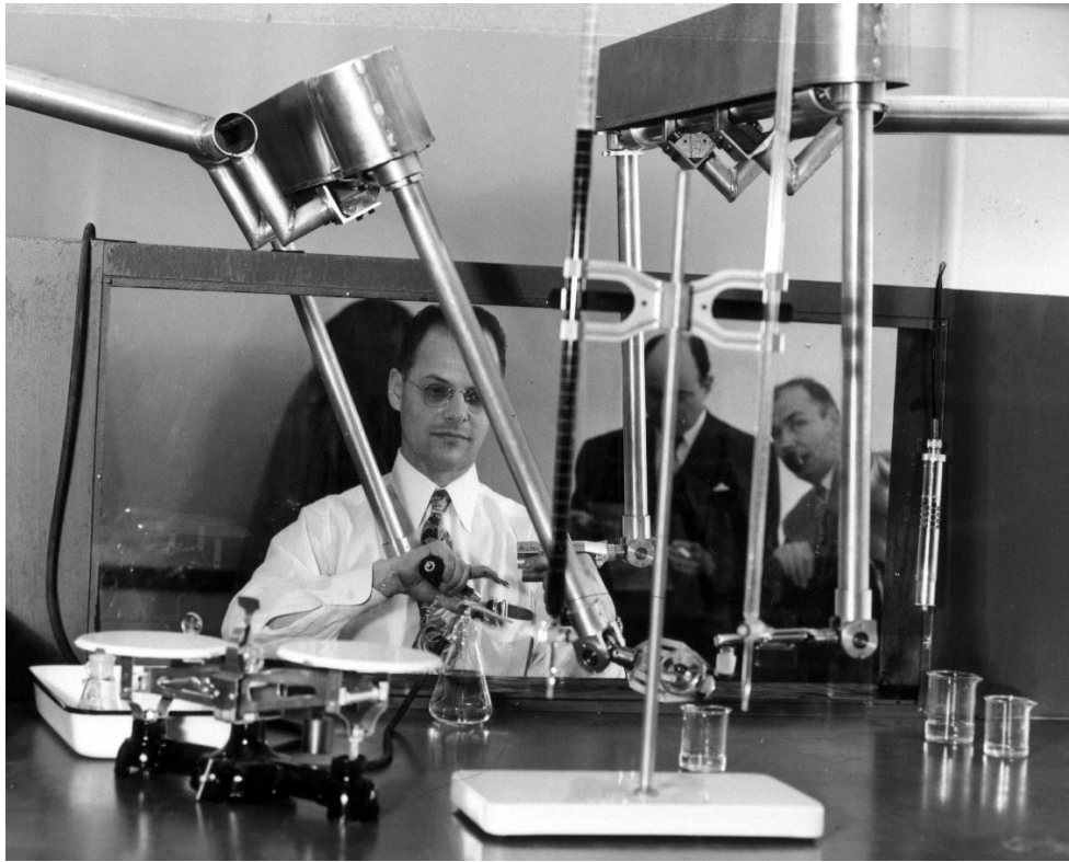
Figure 1.1 One of the First Small Scale Mechanical Link Teleoperator
