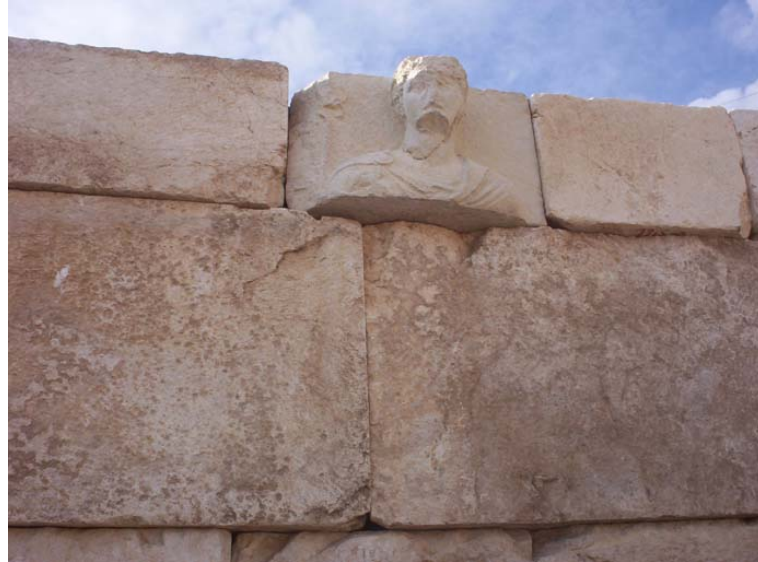
Figure 3.4.1. The topmost stone block bearing the relief of a deity is replaced with the white cement cast on the curved wall of the Lower Agora (author).
