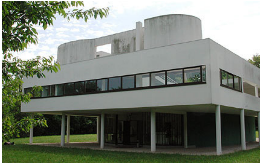
Figure 3.3. Supporting columns and sliding windows of Villa Savoye. 64
