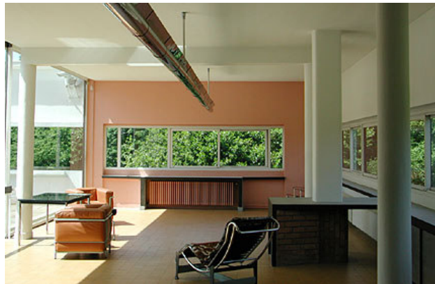
Figure 3.5. Free plan structure of Villa Savoye. 66
