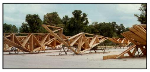
Figure III. 12 Manufactured trusses are stored on site in a proper manner (MiTek Solutions, document on-line).
