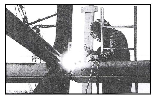
Figure III. 21 Pin welding at the job site (Eggen *et al.*, 1995:43).
