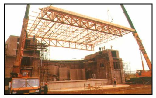
Figure III. 11 25 m x 30 m roof structure over theatre cantilevered off 4 support points. Structure is hold by cranes (MiTek Solutions, document on-line).
