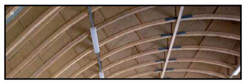
**Figure II. 22** Roof structure of Viikki Teaching and Research Farm<sup>4</sup>; Viikki, Finland (Timber Research and Development Association, document on-line).
