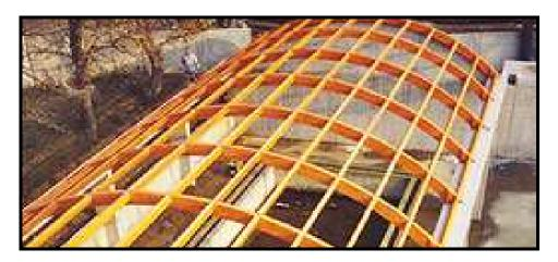
Figure III. 37 Roof structure for the indoor swimming pool of Aytek indoor swimming pool<sup>25</sup> with timber vaults (Oran Mimarlık, document on-line).
