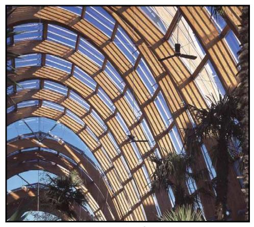
Figure II. 51 Roof structure of Sheffield Winter Garden<sup>9</sup> (MiTek Solutions Catalogue, document on-line).
