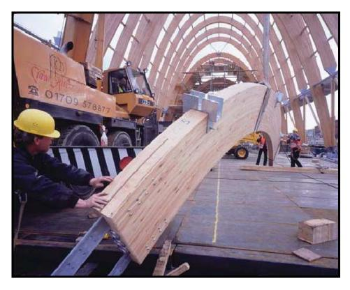
Figure III. 13 Glulam arch with metal connectors at end is being hosted for assembly (Timber Research and Development Association, document on-line).
