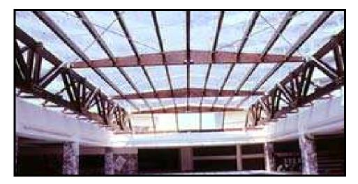
Figure III. 36 Roof structure for the indoor swimming pool of Lares Hotel<sup>24</sup> with timber trusses (Oran Mimarlık, document on-line).
