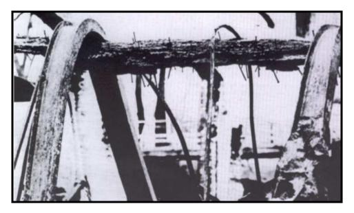
Figure III. 31 Steel beams have melted and collapsed over charred glulam beam which, despite heavy damage, remains in place (Glued Laminated Timber Association, document on-line).
