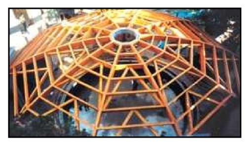
Figure III. 35 Dome structure for the indoor swimming pool of Silyum Hotel<sup>23</sup> (Oran Mimarlık, document on-line).
