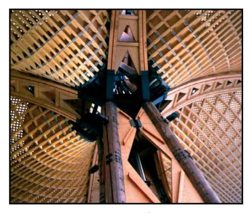
**Figure II. 53** Roof structure of the Hanover Expo Canopy<sup>10</sup>; Hanover, Germany (Timber Research and Development Association, document on-line).
