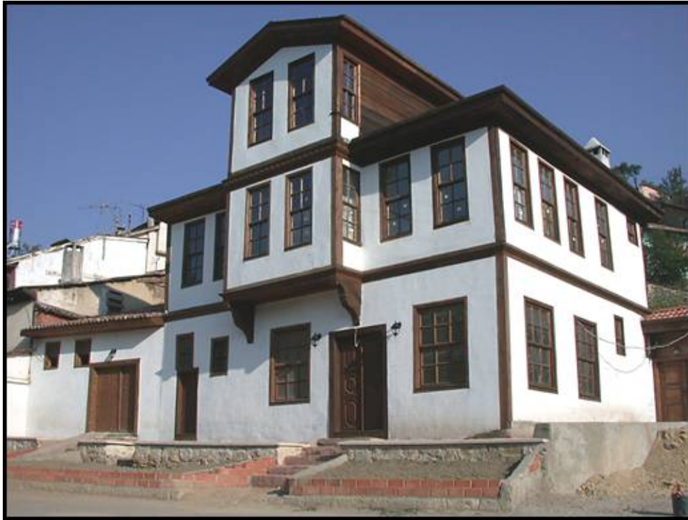
D4. Picture of Toprakçılar House
