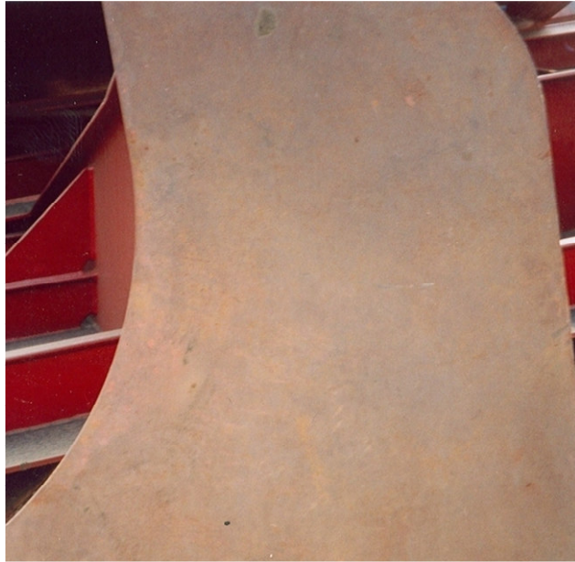
Figure 22: Second Steel Plate before Blast Cleaning
