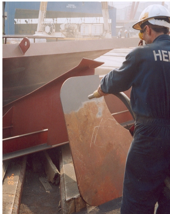
Figure 18: Blasting Operation Using CS
