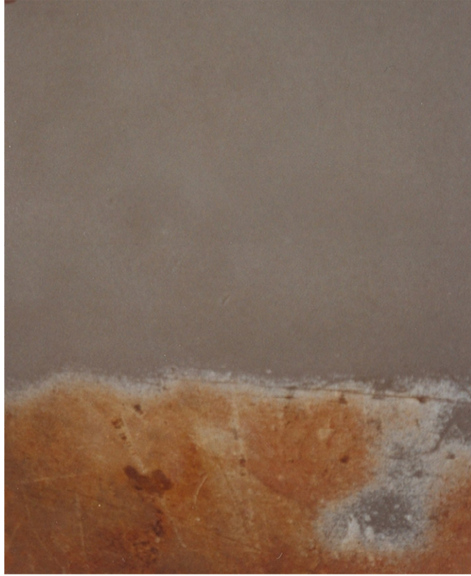
Figure 19: Steel Plate Blasted with CS
