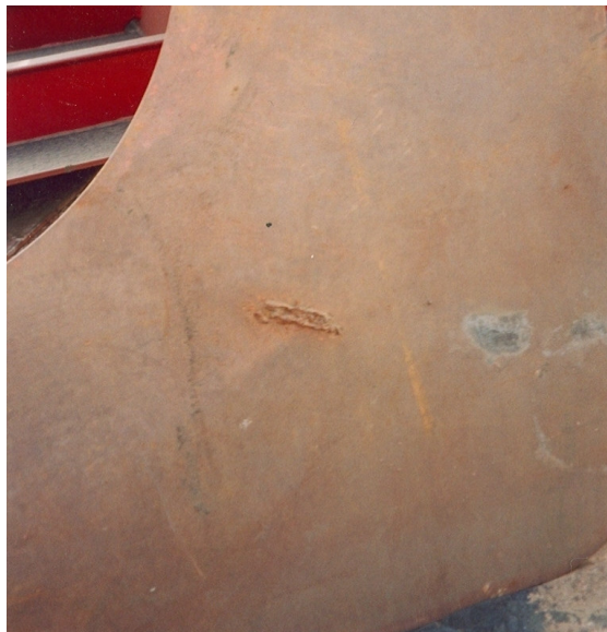
Figure 26: Second Steel Plate before Blast Cleaning
