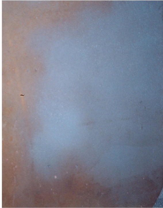
Figure 27: Steel Plate Blasted with CFS
