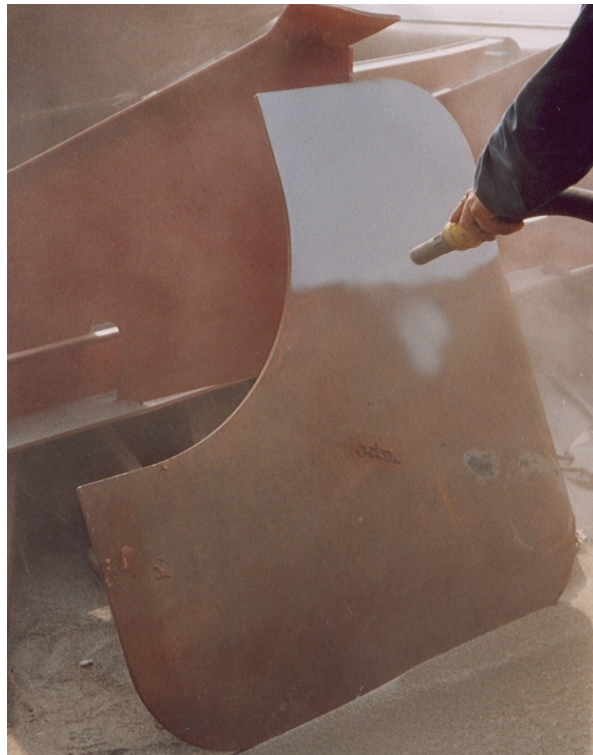
Figure 23: Blasting Operation with Fine GBFS
