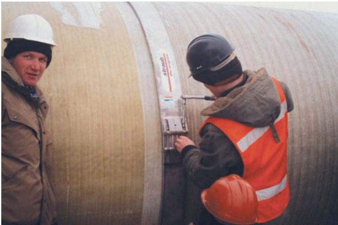
Figure 3.7 Connection of GRP Pipes ( www.superlit.com )
