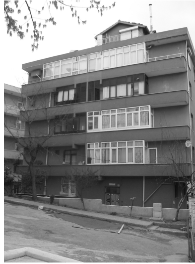
Figure 3.22. Building 4 in Osmaniye
