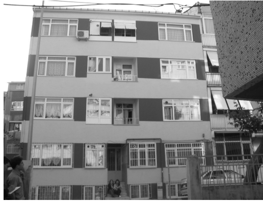
Figure 3.18. Building 3 in Osmaniye
