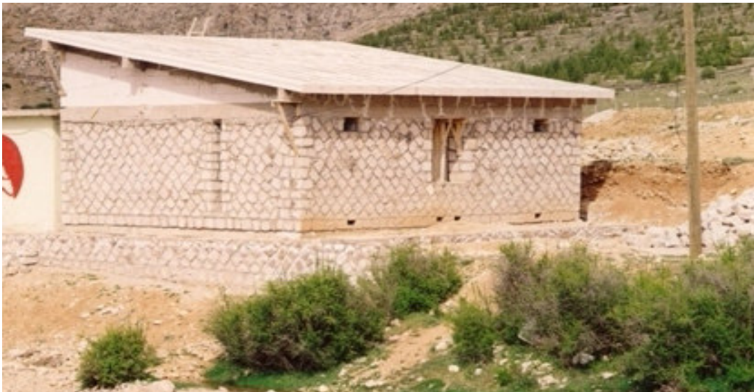
Figure 3.10 Additional Building to Ordos Mountain House, Demirkazık-Niğde (2002)
