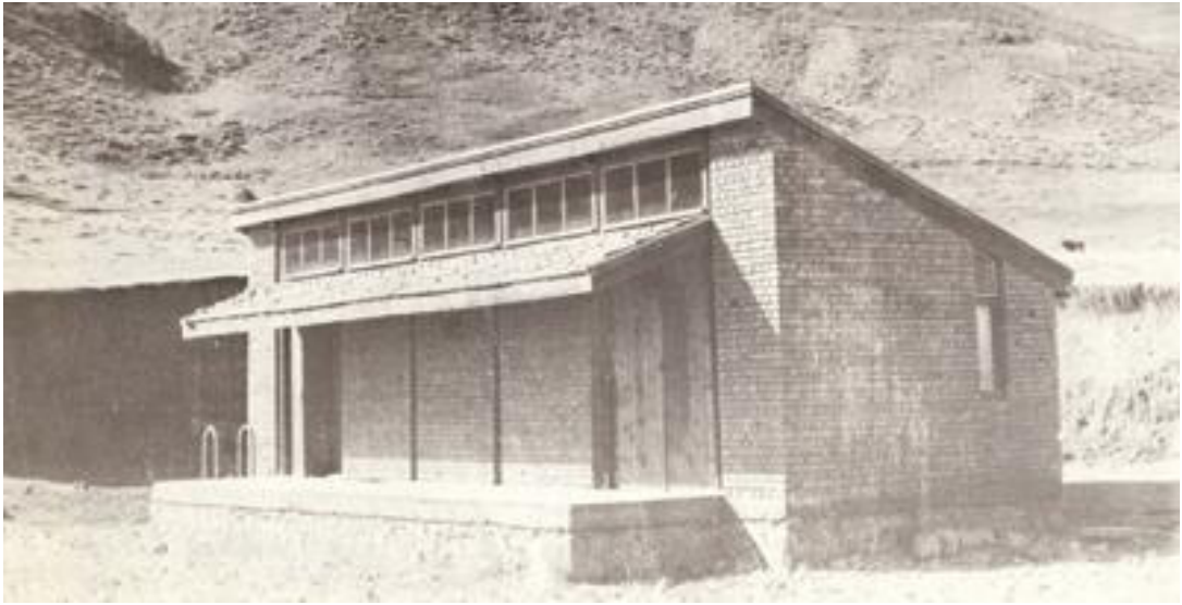
Figure 4.1 Building to bottle spring water Ilca-Sivas (1970)
