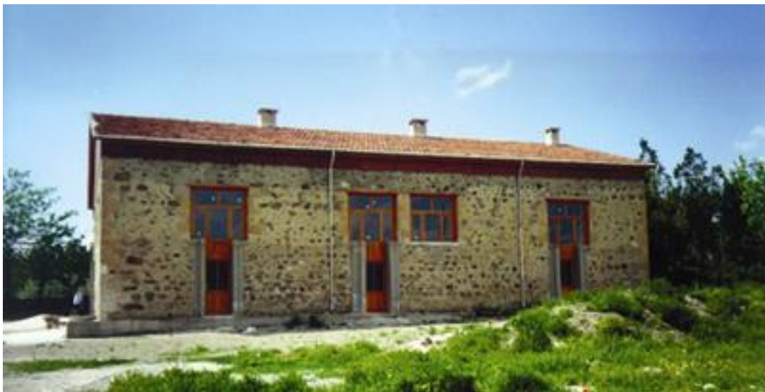
Figure 3.5 Multifunctional Building, Eminlik-Niğde (1999)
