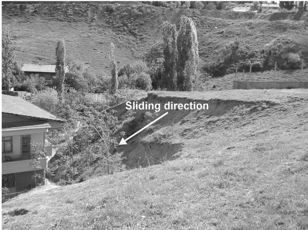
Figure 3.12 General profile of the highly weathered andesites in Ankara and a shallow slope failure occurred within the intensely weathered rock mass.
