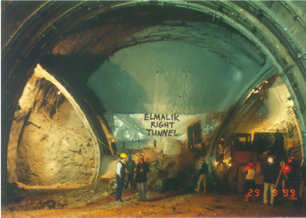
Figure 4.2 Construction of Option 4 (Yüksel Proje, 1999)
