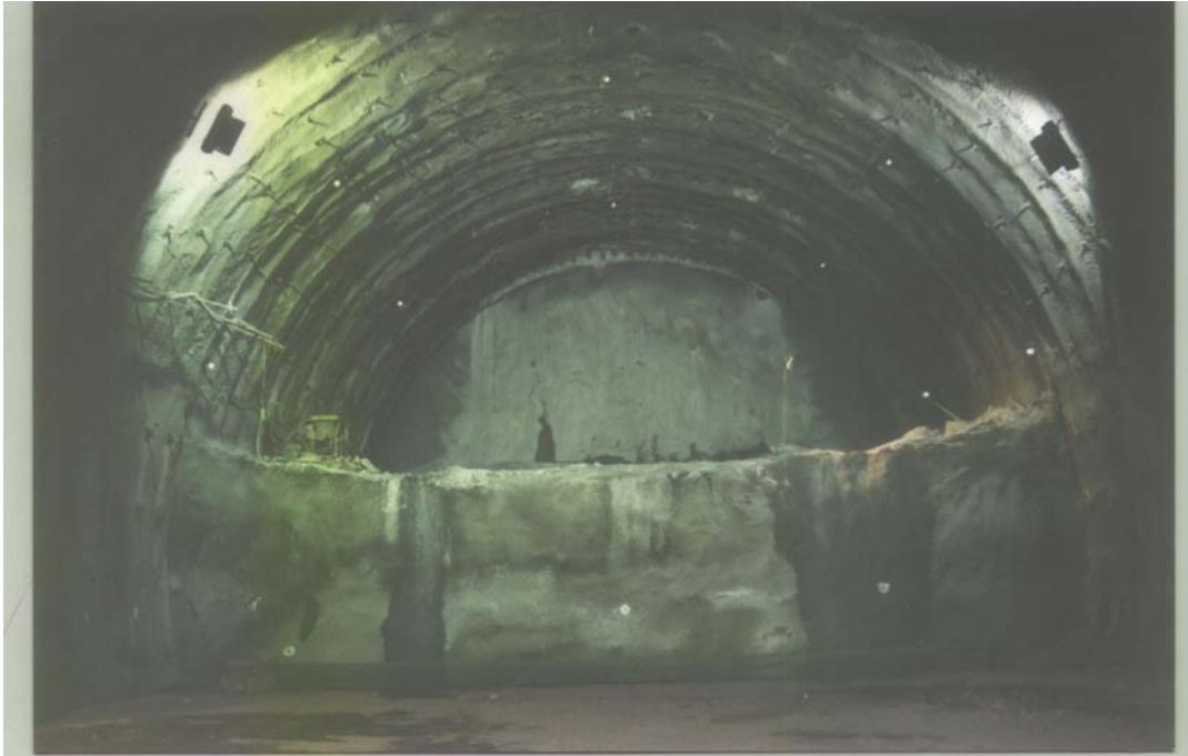
Figure 4.3 Staged excavation for Option 4 (Yüksel Proje, 2003)
