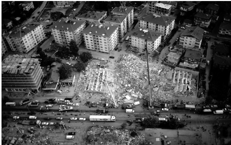
Figure 1.1 Air photo after 17 August 1999 Kocaeli Earthquake (courtesy of, METU-GISAM)
