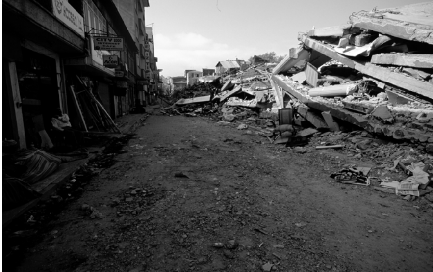
Figure 1.2 Almost fully collapsed avenue during 17 August Kocaeli Earthquake (courtesy of, METU–GISAM)
