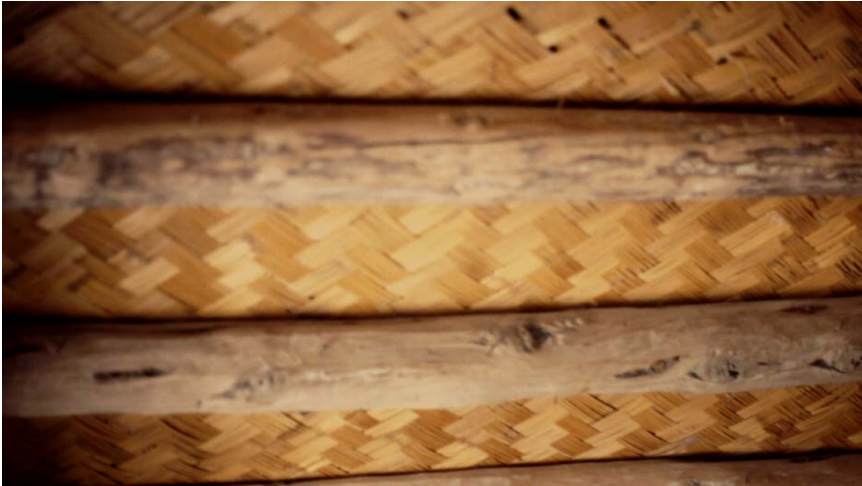
Fig. 5. Club rush stems used on the ceiling.
