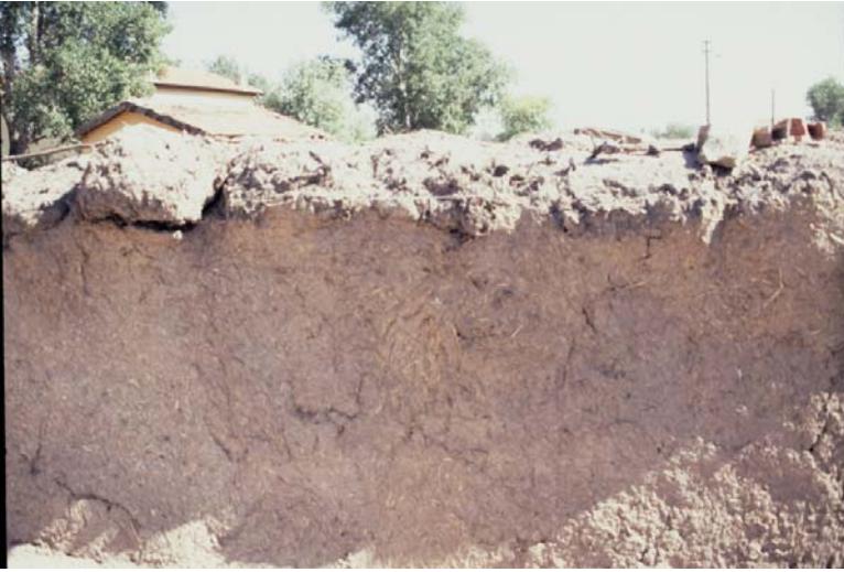
Fig. 7. Scirpus maritimus used in and on mudbrick wall.
