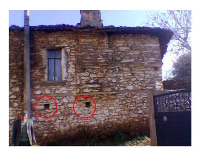
Figure 154, A dwelling in Hacı Arap Street, Karşıyaka, exterior wall with ventilation niches (Taşdöğen)
