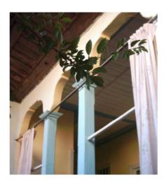
Figure 132, Timber colonnades with Bursa-type arches in *hayats* of a demolished dwelling and Case 1 (Taşdöğen)
