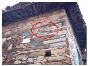
Figure 155, Corner details created with stone in Karşıyaka (Taşdöğen)
