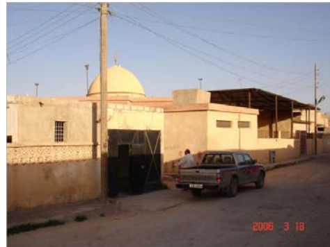
Figure 5.53: Ain Jaloot Mosque, General View
