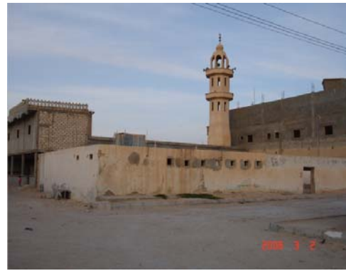
Figure 5.26: General View of Ghazwat Honain Mosque
