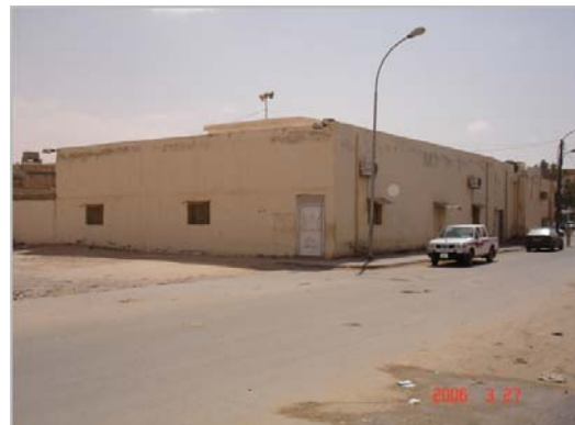
Figure 5.8: An Outdoor View of al-Ansar Mosque
