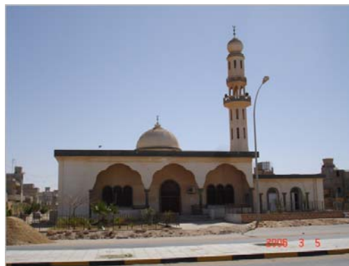
Figure 5.69: Al-Taneem Mosque, General View
