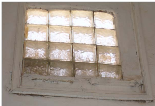
Figure 5.55: Bay'at al-Raddwan Mosque, Canceled Window
