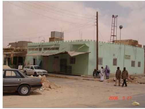
Figure 5.43: Al-Qadesya Mosque, an Exterior View
