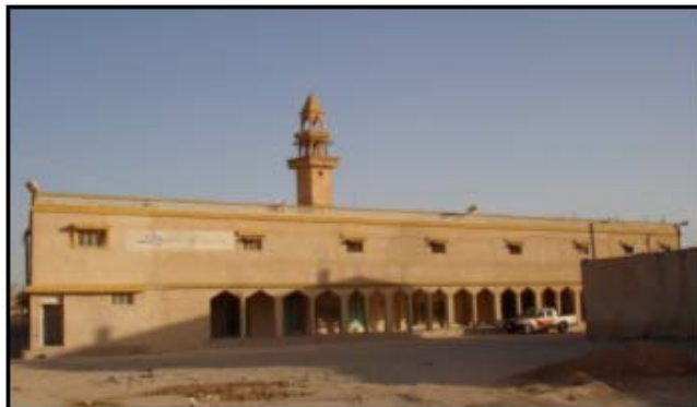
Figure 5.33: Teboak Mosque, Main Elevation
