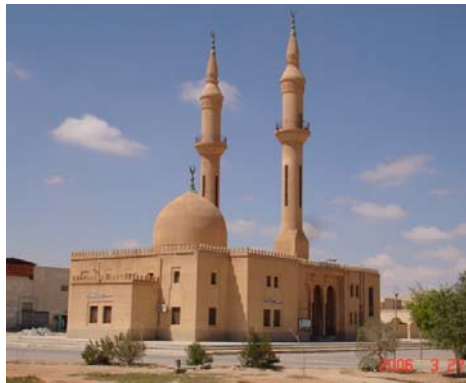
Figure 5.28: Al-Esra Mosque, an Outdoor View
