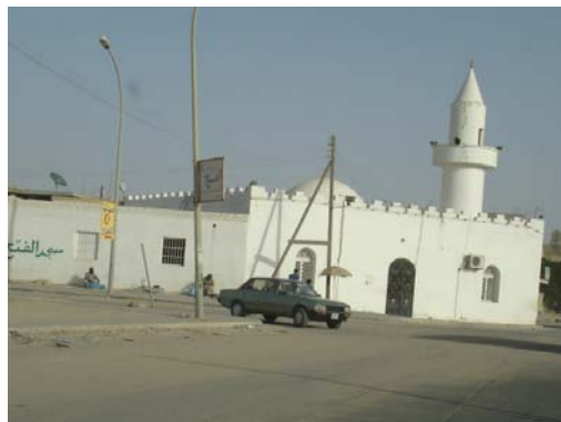
Figure 5.17: Al-Fatah Mosque, An exterior View
