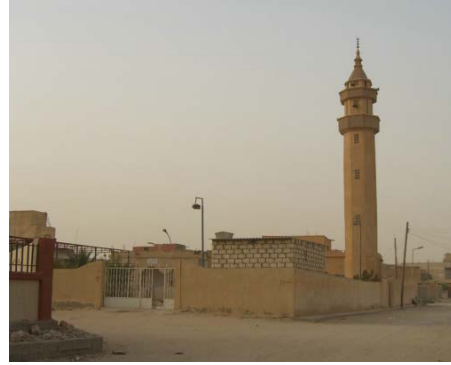
Figure 5.62: Hetteen Mosque, Disproportionate Minaret
