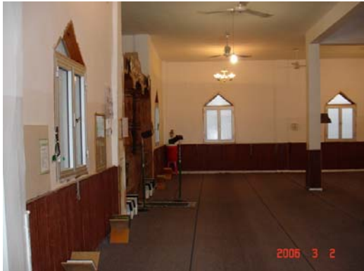
Figure 5.121: Al-Er'wa al-Wethka Mosque, Poor Illumination
