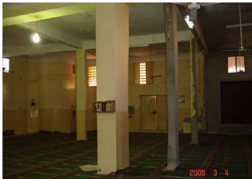
Figure 5.10: Ammouria Mosque, Poor Illumination, Improper Size and Form of Columns
