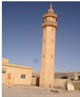
Figure 5.63: Hetteen Mosque, Disproportionate Minaret
