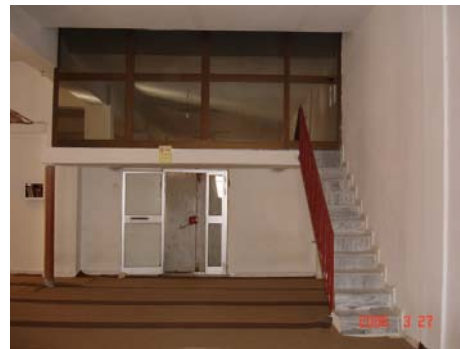
Figure 5.104: Bab al-Marwuha Mosque, Unused Room
