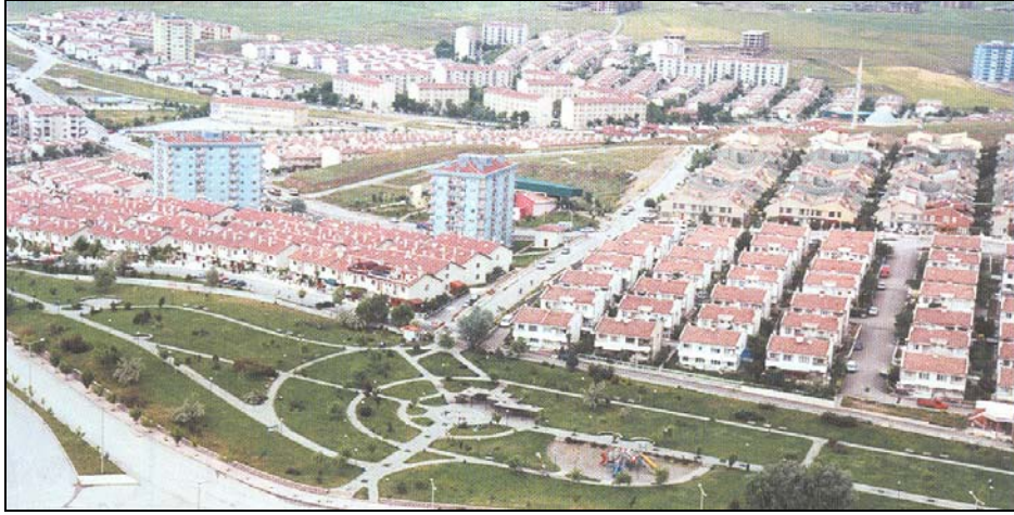
Figure 5. 8: Aerial view of Batkent
