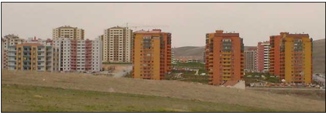
Figure 6. 23: High-rise Blocks in Yenikent
