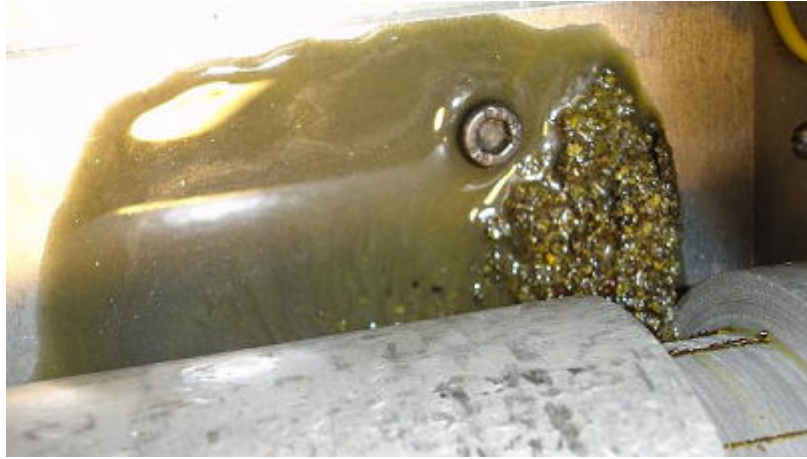
Figure 5.9: View of the recovered oil after the failure
