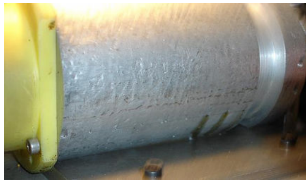
Figure 5.8: View of oil leaking out from the vessel
