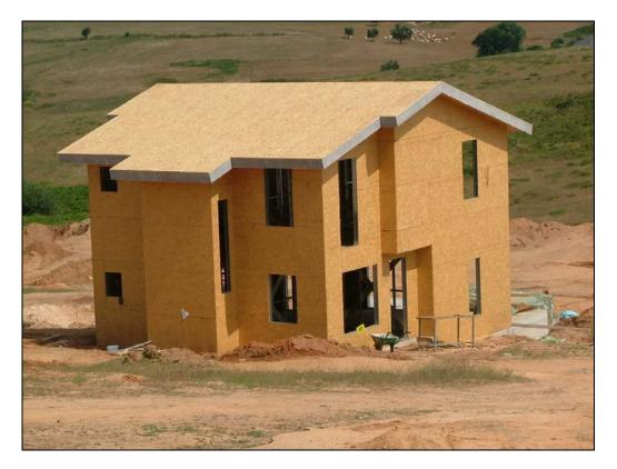
Figure 3.1 OSB Sheathed Light Gauge Steel House.
