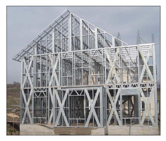
Figure 1.7 Shear Walls with X-bracing on a light gauge steel house
