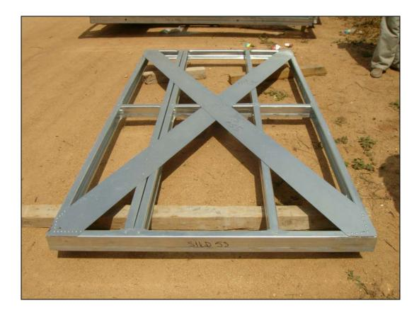
Figure 5.2 Frame with X-bracing
