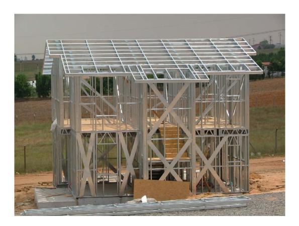
Figure 1.1 Steel frame of a light gauge steel house
