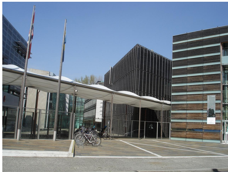
Figure 3.11 “The Platz” as an extension of the urban public space, Berlin, 2006 (Photography; by the author).
