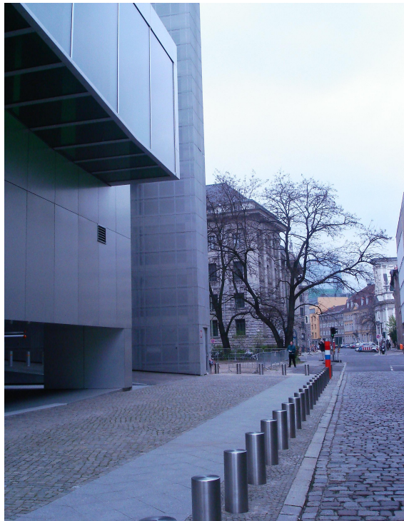
Figure 2.1 The determination of the Dutch Territory within public realm. The architecture of the boundary (interpreted as cylindrical objects placed scattered), separating the private from the public realm, allows public intrusion within the Dutch Territory, the Dutch Embassy in Berlin, 2006 (photography; by the author).
