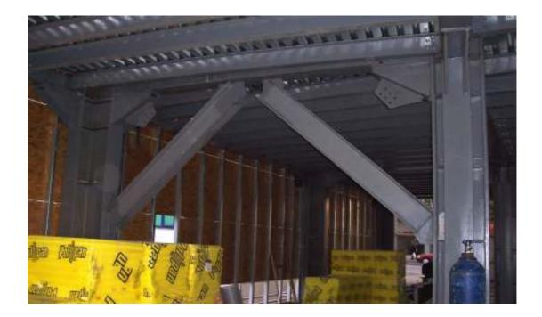
Figure 4.32. Rectified structural bracing
