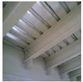
Figure 4.14. A plate welded to the beam for the girders
