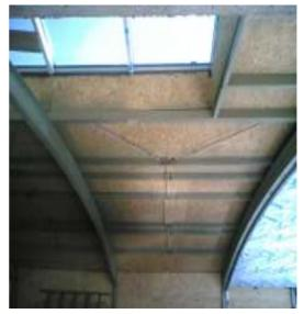
Figure 4.8. Curved steel beams
