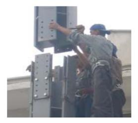
Figure 4.17. Assembly of the columns by using splice plates
