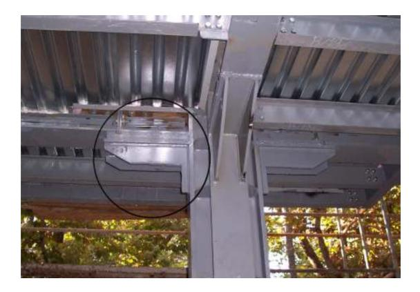
Figure 4.33. The modification made on gussets
