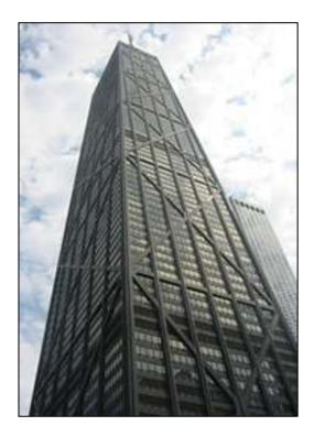
**Figure 2.12.** Use of external steel bracings in the John Hancock Center in Chicago, USA (Source: www.hispago.com, retrieved 2006)
