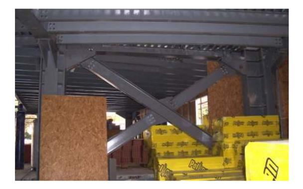
Figure 4.31. Incorrect structural bracing
