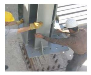
Figure 4.16. Anchorage of the columns to the concrete plinth
