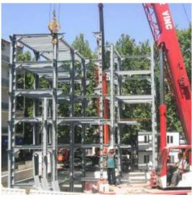
Figure 4.18. Assembly of the columns
