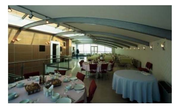
Figure 4.37. Curved beams supporting the roof
