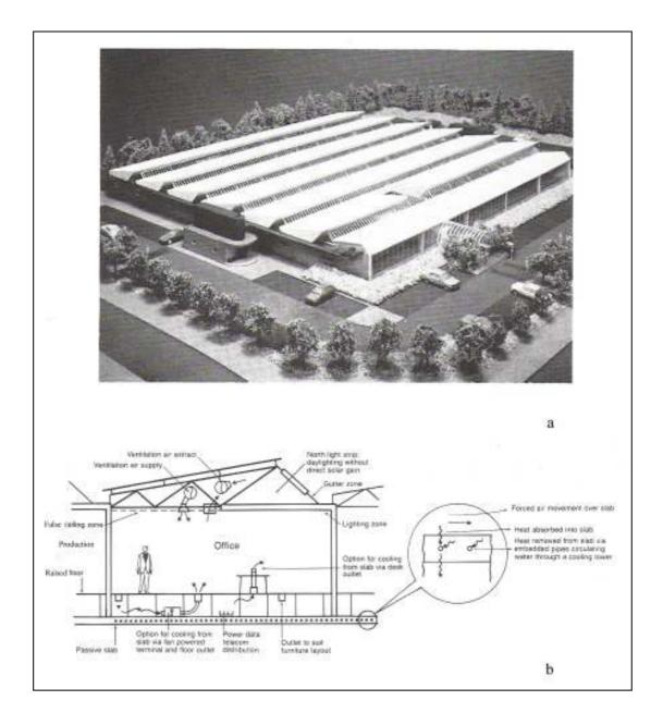
Figure 2.27. Spectrum 7 Building, Milton Keynes, UK; (a) photo, (b) cross-section (Source: Plank, 1993)
