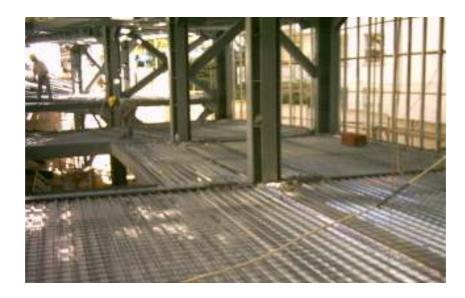
Figure 4.9. The construction of metal deck floor
