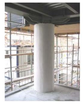
Figure 4.24. The steel column and the installation channel enclosed within gypsum board casing
