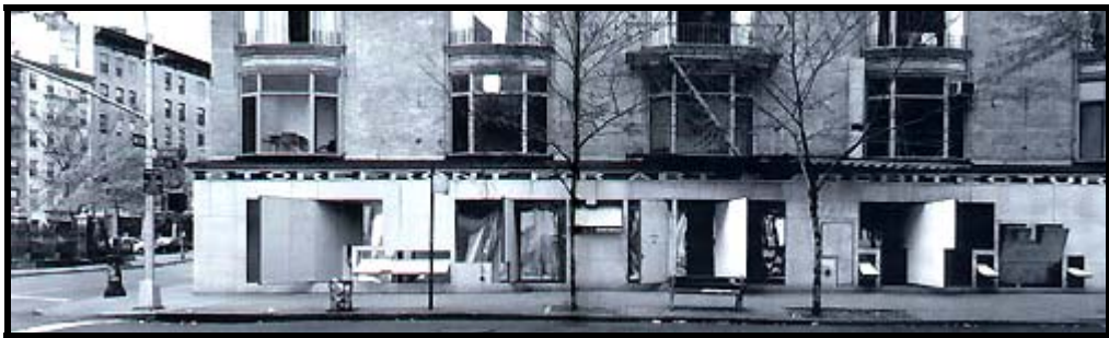
Figure 4.1 and 4.2: Exterior views of Storefront for Art and Architecture when it is open and closed.
