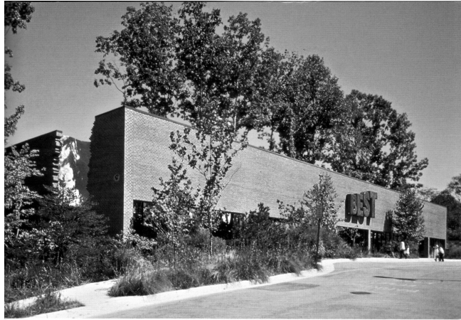
Fig. 4.31. SITE, Best Forest Building, Richmond, Virginia, USA, 1980.
