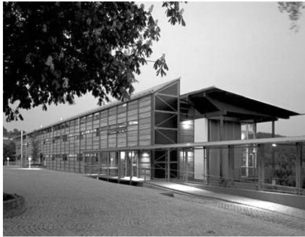
Fig. 4.7. Thomas Herzog , Guest Building for the Youth Educational Centre in Windberg, Germany , 1987-1991.
