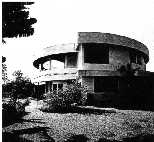
Fig. 4.25. Ken Yeang, Ulysees House, Kuala Lumpur, 1976.
