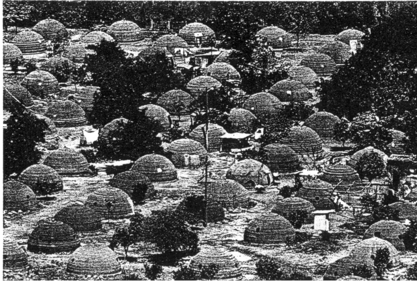
Fig. 3.33. Papanek's example on the vernacular: "Foam domes, post-earthquake emergency shelters of polyurethane, 1972, Nicaragua."
