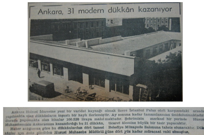
Figure 29a, Construction of new shops in Ulus commercial area, Ulus 23 7 1943
