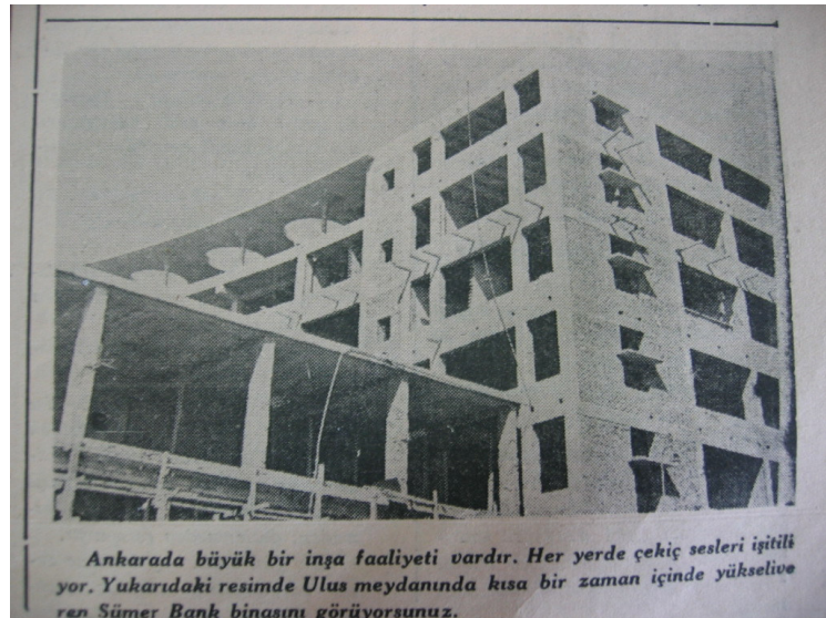
Figure 16b, Sümerbank under construction, Ulus: 28 8 1937
