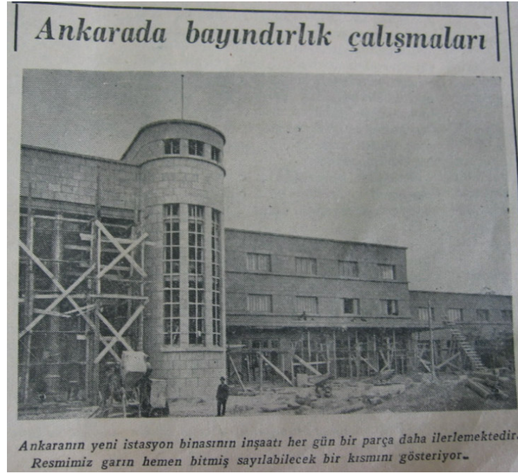
Figure 17, The Train Station, under Construction, Ulus: 13 5 1937
