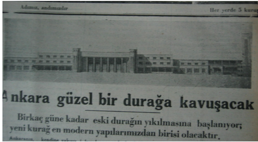
Figure 13, The new train station, Ulus: 17 7 1935
