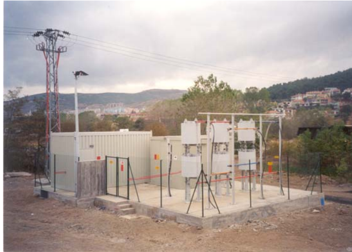
Figure 1.3 SVC-Thyristor Controlled Reactor
