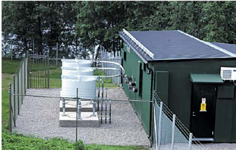
Figure 1.6 Voltage Source Converter Based STATCOM
