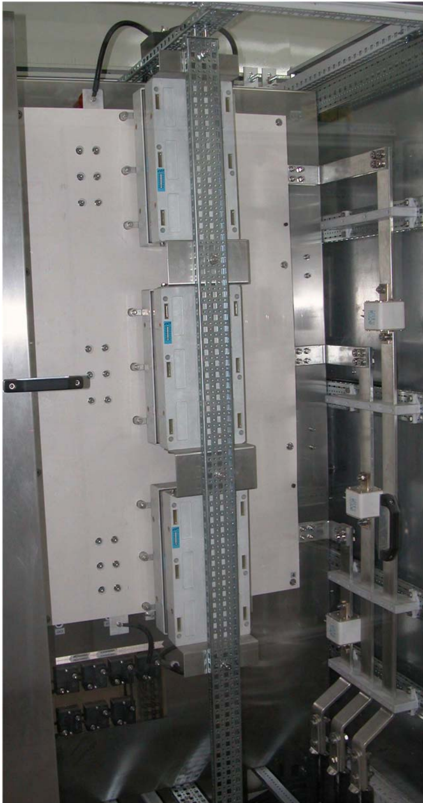
Figure 3.48 DC Link Capacitor Placement in VSC
