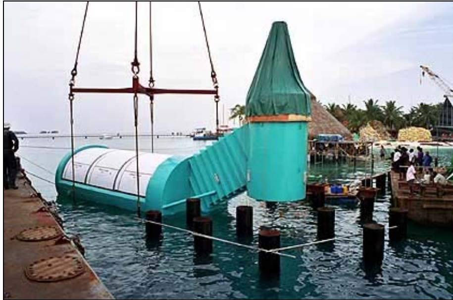
Figure 40. Placement of the structure.
