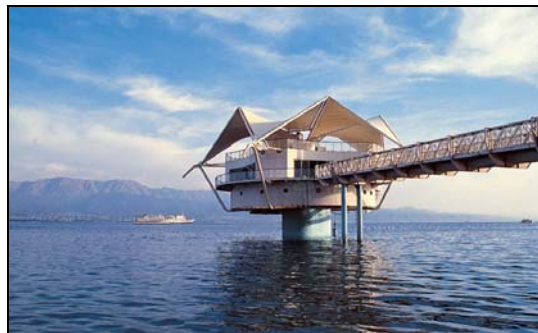
Figure 44. Restaurant is entered through a bridge and staircase.
