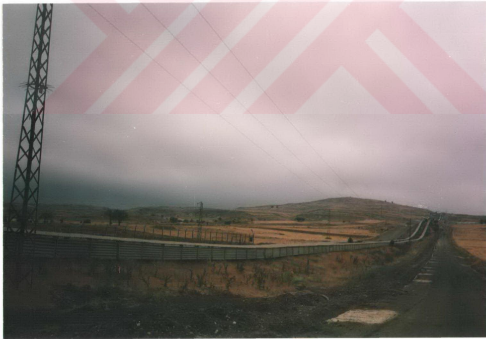
Figure 3.7. Photograph of conveyor belts for solid waste transportation from plant to the disposal site
