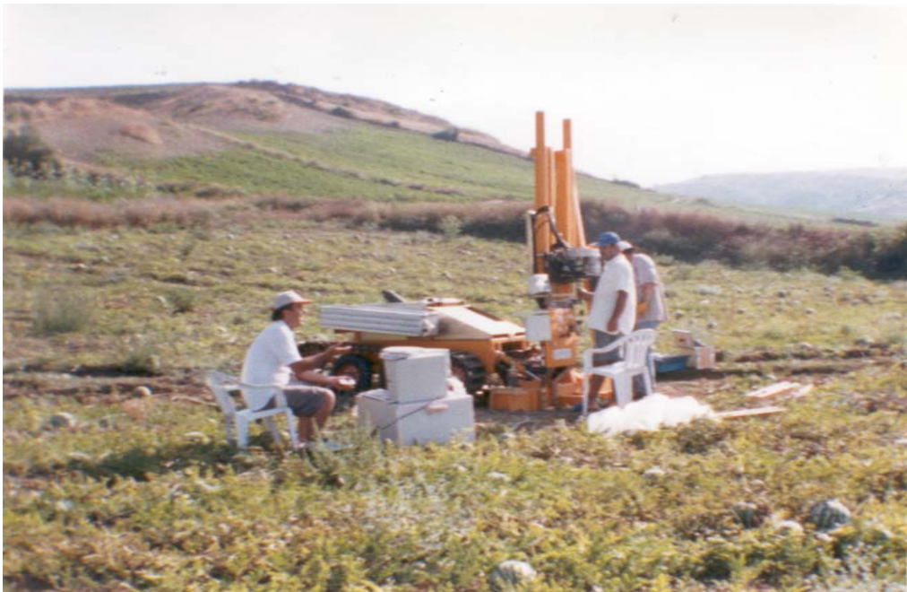
Figure 2.4 A Penetration Type In-Situ Test Work on Field (CPT)
