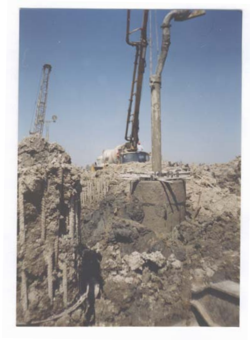
Figure 3.14 Gray colored silty clay deposits of İzmir Alluviums extracted during a bored-pile excavation
