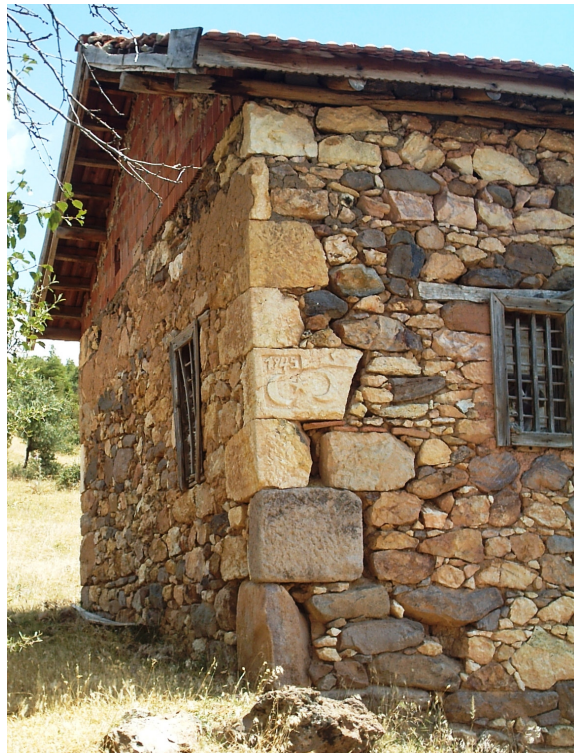
Figure 4.7 Structure built with undressed stone and dressed stones at corners using clay mortar in 1945 at Katrancılar District
