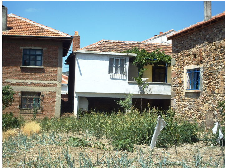
Figure 4.11 Different structure types at Gümüşkol Village; rubble stone building with clay mortar at right, lime mortared solid/cellular brick walled and reinforced but not engineered structures at the middle and left
