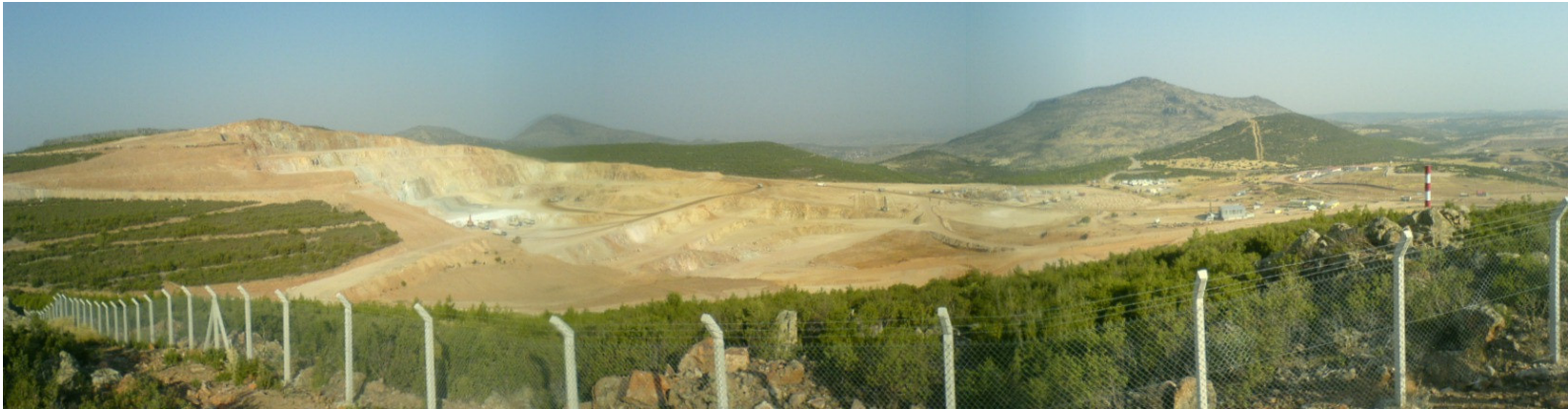
Figure 3.2 General view of Uşak Kışladağ Open Pit Gold Mine from the mine site.
