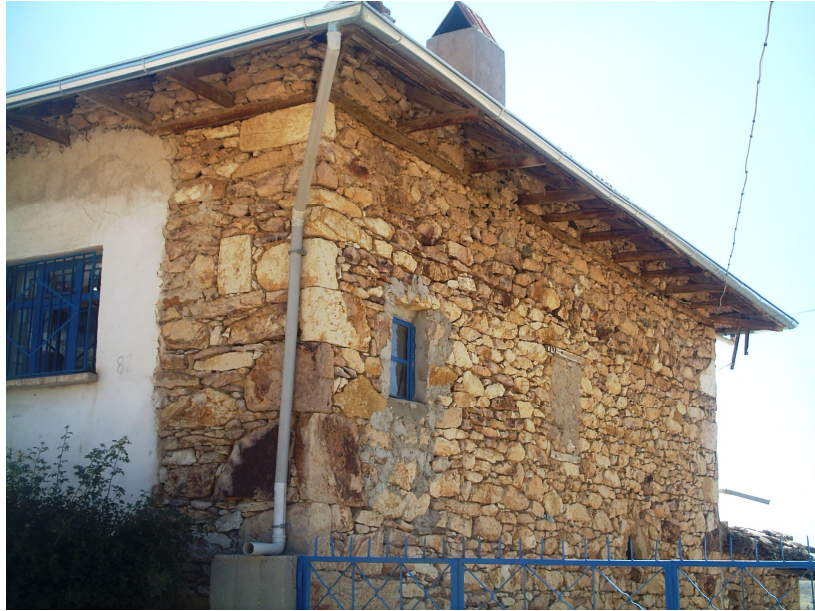
Figure 4.6 Clay mortared rubble stone building at Gümüşkol Village
