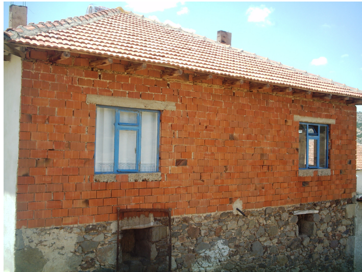
Figure 4.13 Two story hybrid structure at Micanlar District (rubble stone wall at ground floor and cellular brick wall at first floor are laid using clay mortar, lintels above windows are reinforced concrete)
