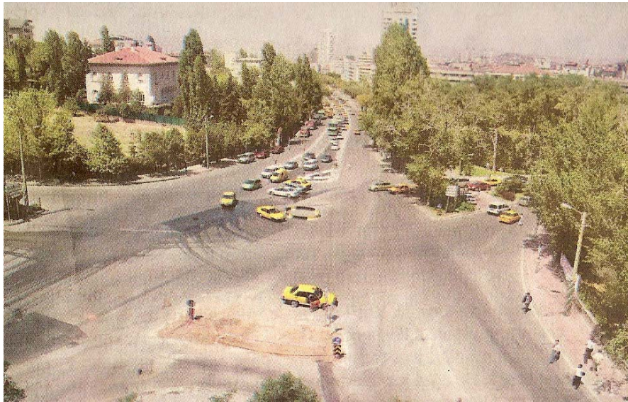
Figure 3.2: Existing situation of Kuğulu Intersection (Ankara Büyükşehir Belediyesi, 2006)
