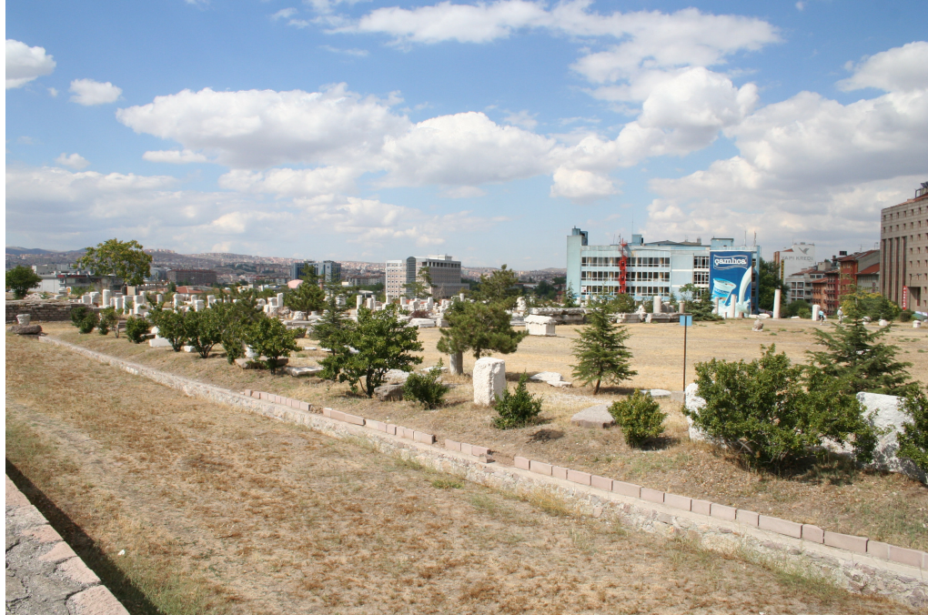
Figure 3. 19 The palaestra , view from north, The Caracallan Bath-Gymnasium Complex at Ankara (Photo: Oya Dinler)
