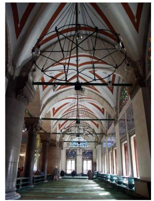
**Figure 109** The cross-vaulted side galleries of the Kılıç Ali Pasha Mosque. Photograph by C. Katipoğlu, 2006.
