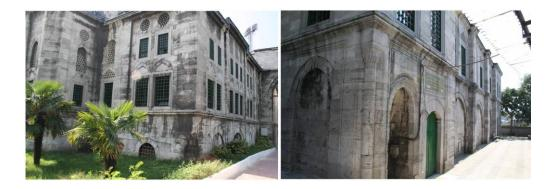
**Figure 27** Left: South and east vaulted stores on the basement level of the mosque. Right: North vaulted stores on the basement level of the mosque. Today these shops are buried due to a recent renovation. Photographs by C. Katipoglu, 2006.
