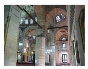
**Figure 40** The arches of the octagonal baldachine and the buttresses carried the upper galleries. Photograph by C. Katipoglu, 2006.
