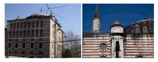
**Figure 121** Left: the south (mihrab side) and west façade of the Şahsultan and Zal Pasha Mosque. Right: the detail of the buttress and waterspouts on the south façade of the mosque. Photographs by C. Katipoğlu, 2006.
