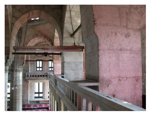
**Figure 42** The arches of the Azapkapı Mosque which tie to the buttresses and pillars. Photograph by C. Katipoglu, 2006.
