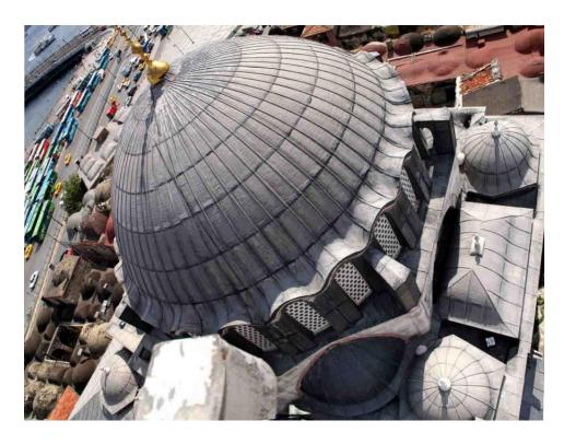
**Figure 17** One vault and two dome cover of the west wings of the mosque. Photograph by C. Katipoğlu, 2006.
