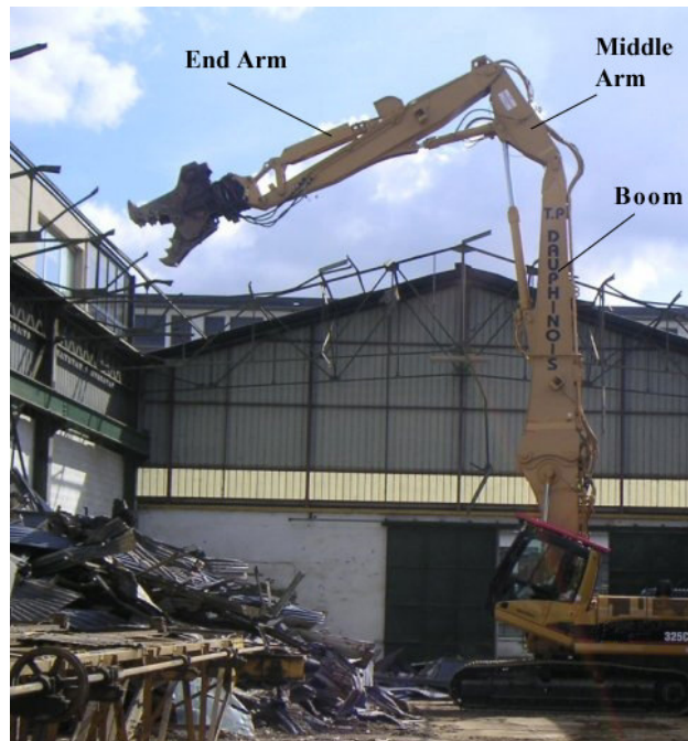
Figure 1.5: A demolition excavator
