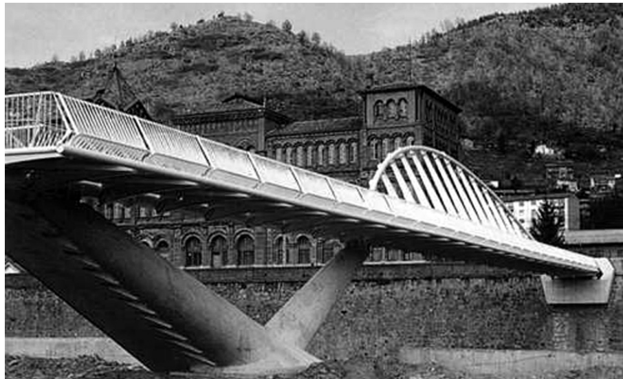
Figure 4-5 La Devesa Footbridge
