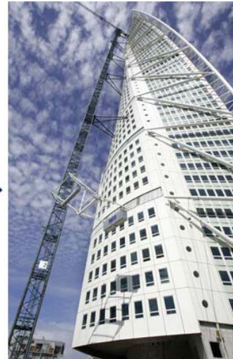
Figure 4-20 left: High Rise in Malmö _ exemplary floor plans changing angles and core-walls right: High Rise in Malmö _ twisting steel truss
