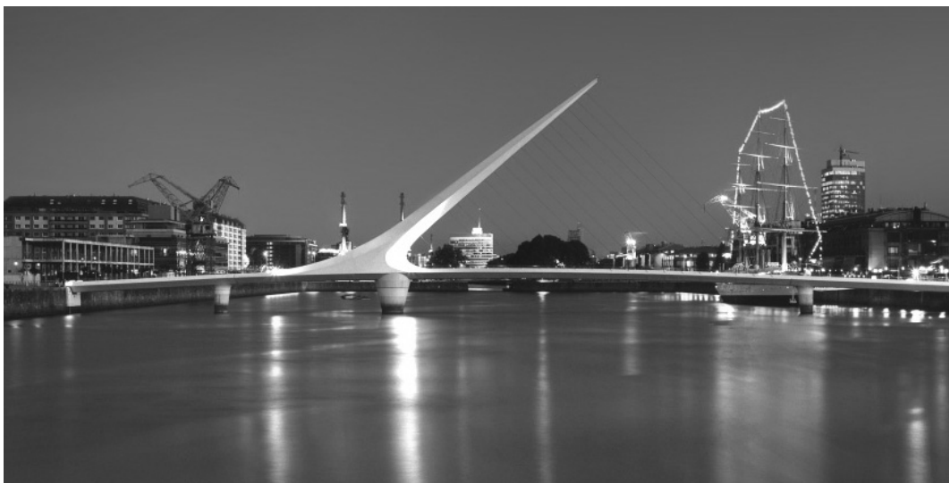
Figure 2-18 Footbridge Puerto Mujer
