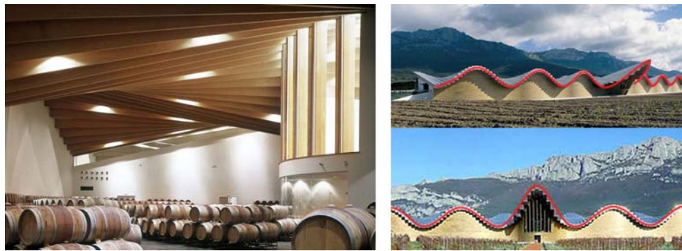
Figure 4-24 left: La Rioja Bodegas Ysios Winery _ interior view right: La Rioja Bodegas Ysios Winery _ captured S-forms
