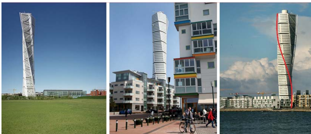
Figure 4-21 left & middle: High Rise in Malmö _ exterior views right: High Rise in Malmö _ captured S-form
