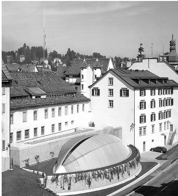
Figure 2-7 Pfalzkeller Emergency Service Center_ exterior view
