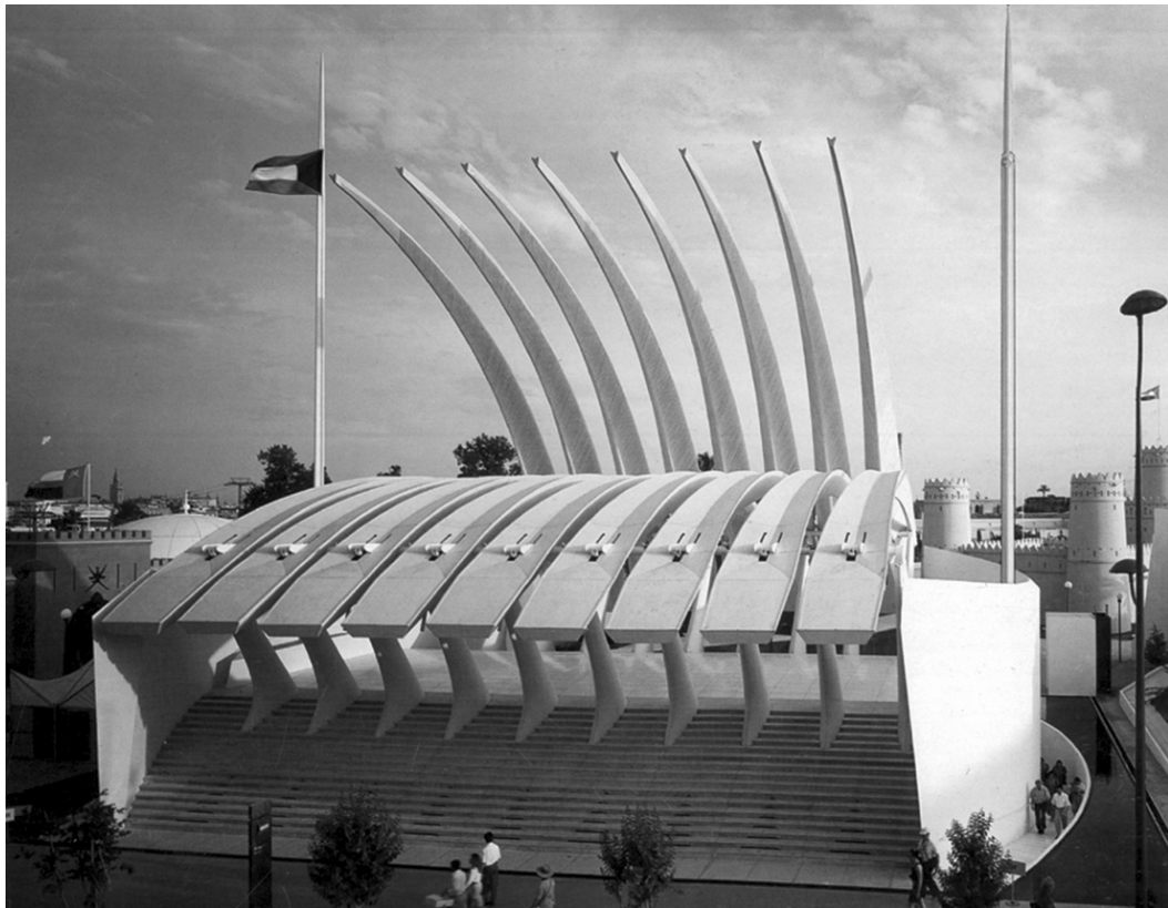
Figure 2-11 Kuwait Pavilion _ exterior view
