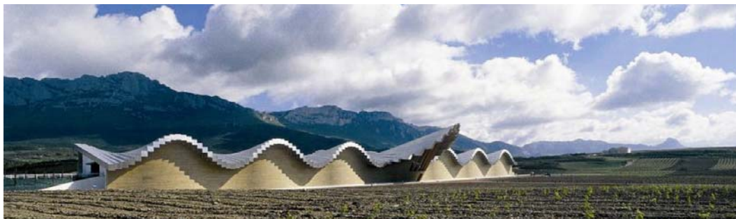
Figure 4-22 La Rioja Bodegas Ysios Winery _ exterior view
