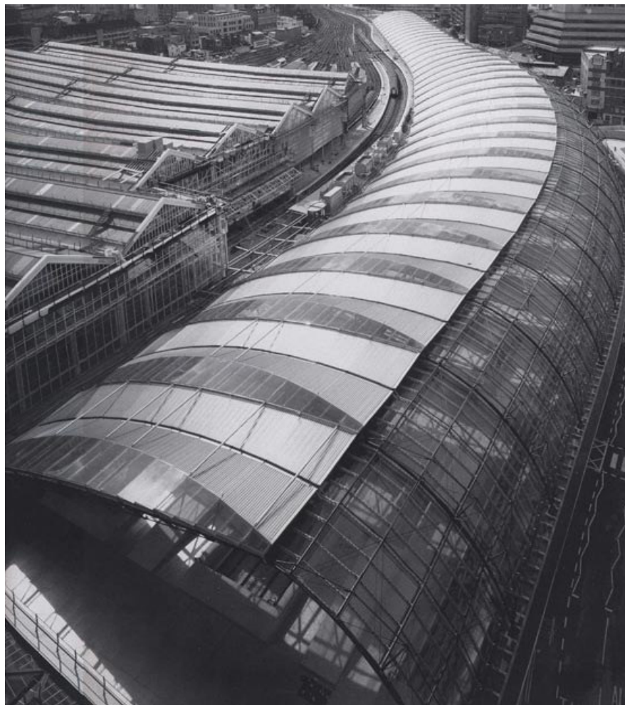
Figure 72. The glazing of the curvilinear roof
