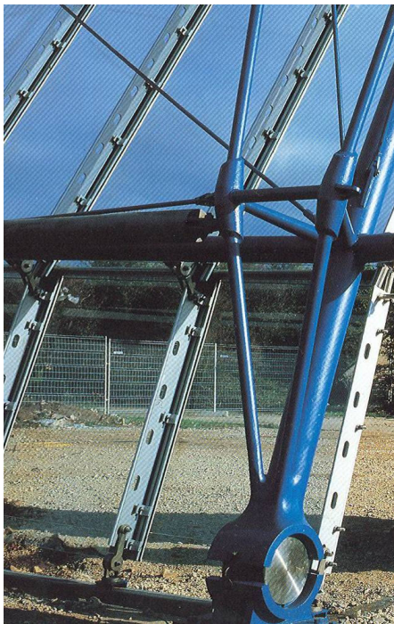
Figure 71. Pin joint detail
