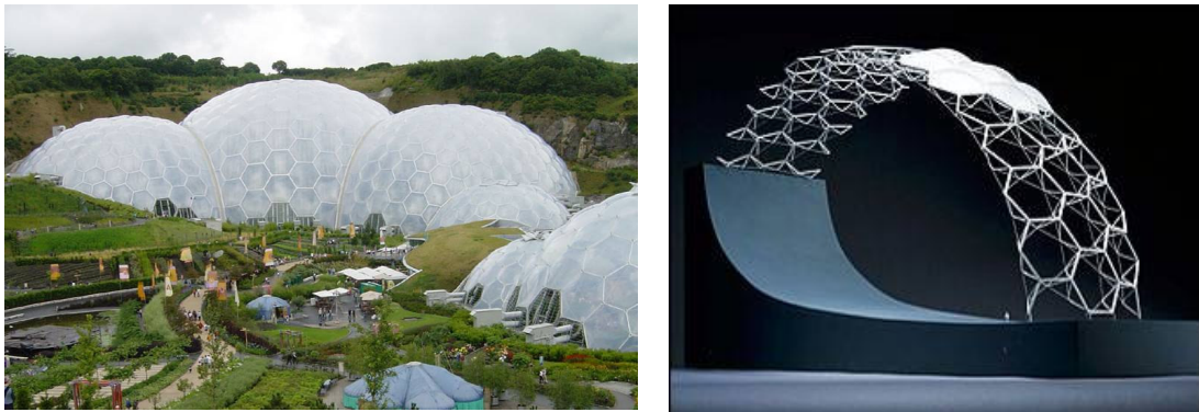
Figure 65. Eden project and section through the dome
