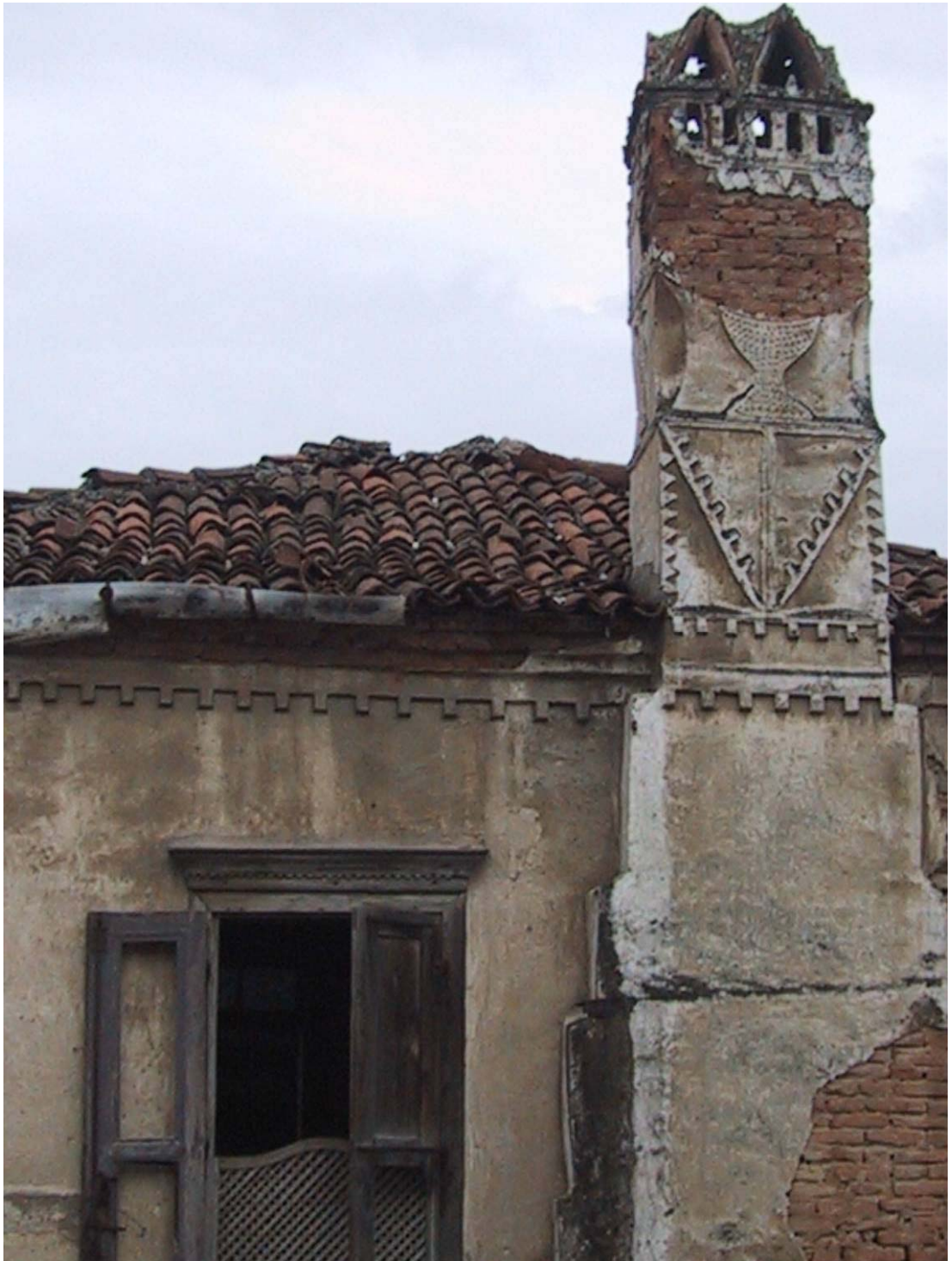
Pl. 56 Traditional chimney of a house in Milas
