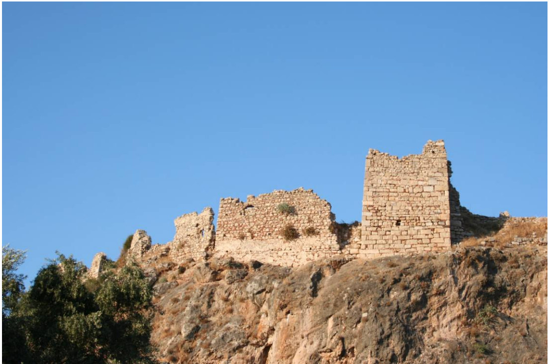
Pl. 7 Beçin Kale, close view of the restored fortifications.
