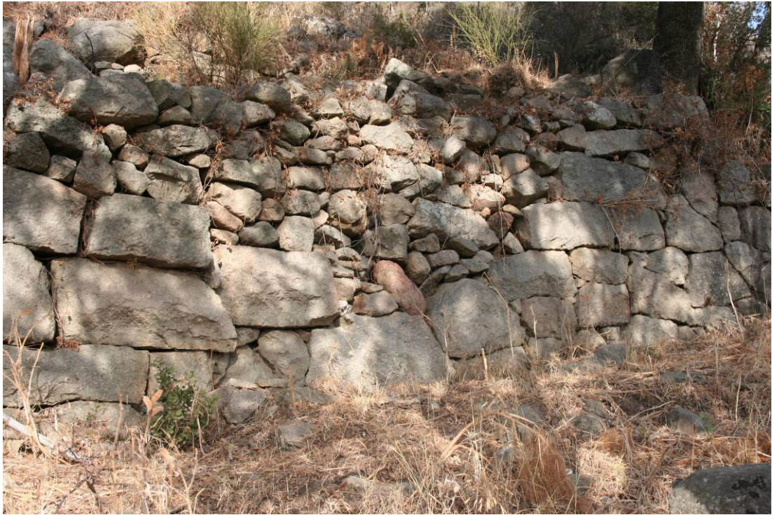
Pl. 4 Polygonal terrace walls over the Lelegian substructure in Geriș, which may have formed the ancient lower city wall. Lelegian masonry can be traced in the lower courses.
