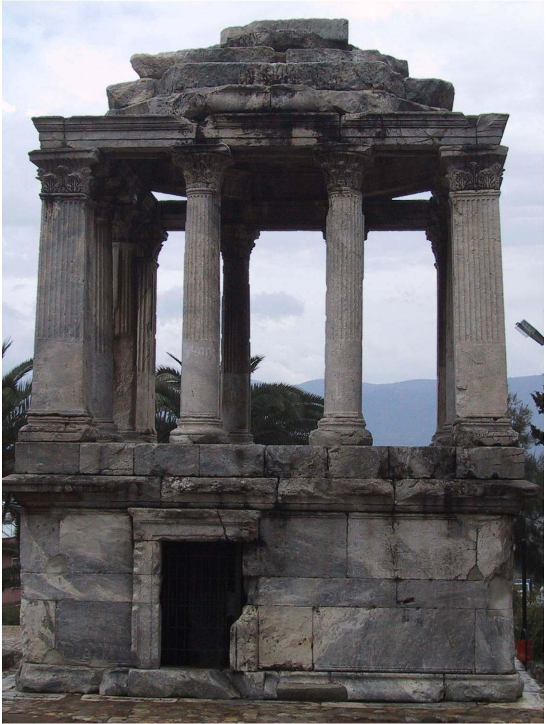
Pl. 53 Gümüşkesen Monument general view
