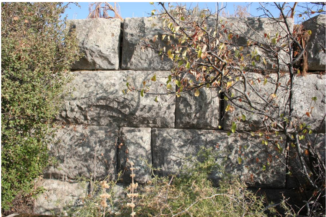
Pl. 3 Fortification (tower) walls in Geriṣ displaying the Hekatomnid masonry technique.
