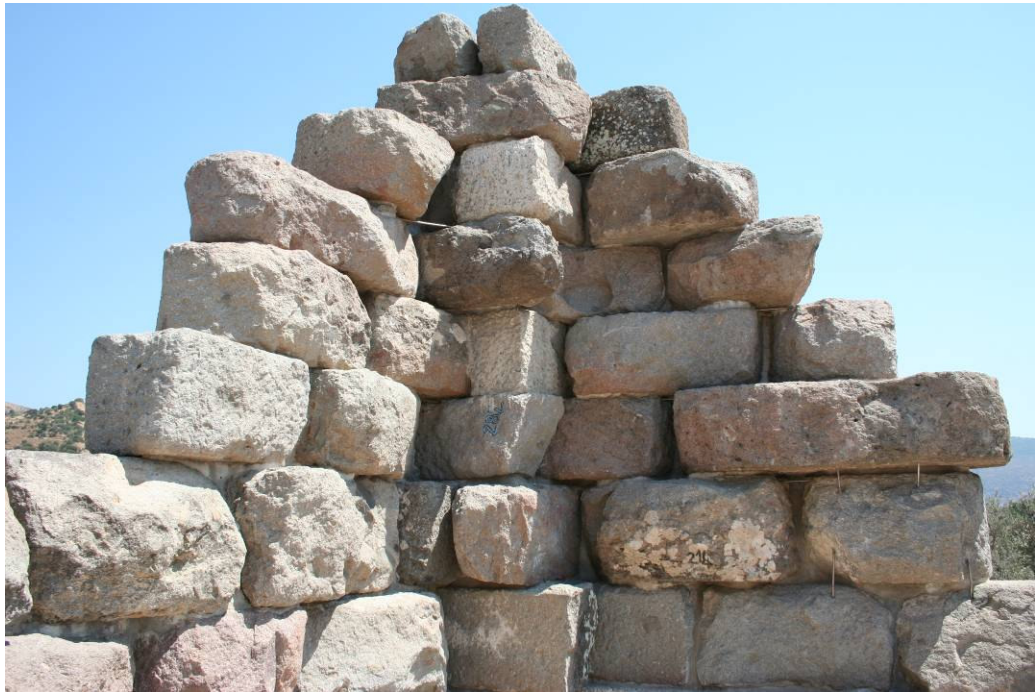
Pl. 10 Myndos Gate details of the masonry technique – interior view.
