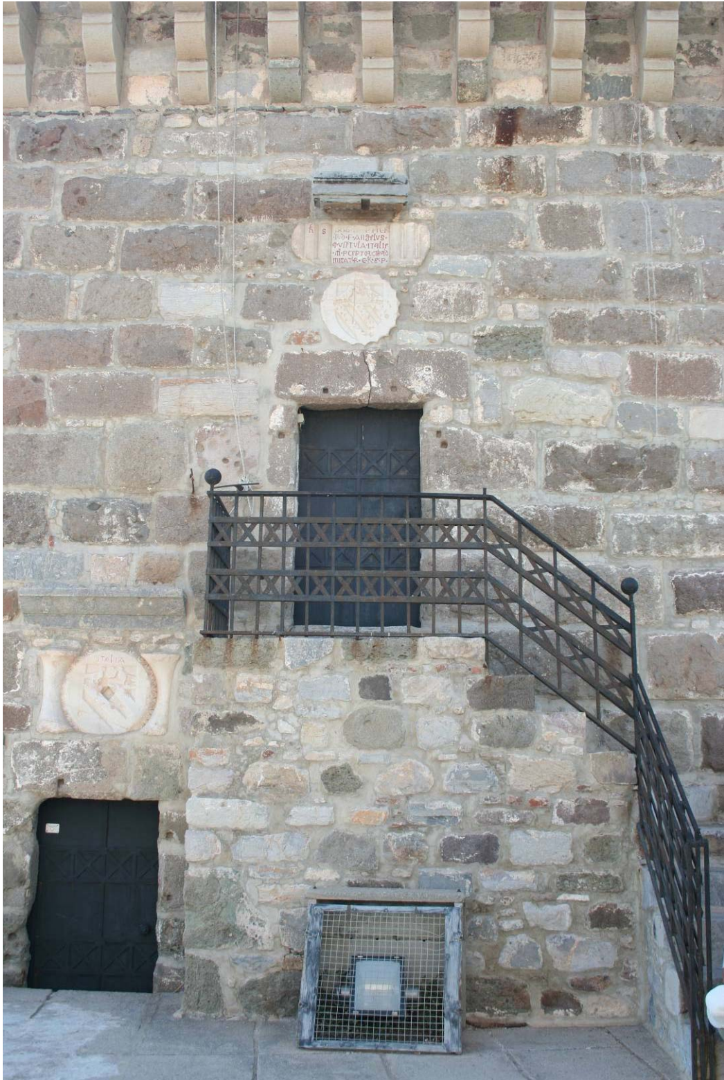
Pl. 46 Reused material derived from Maussoleion and other ancient buildings on the walls of Bodrum Castle
