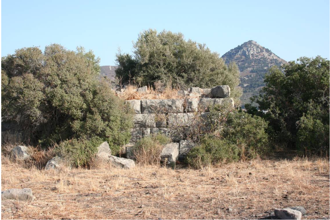
Pl. 2 Close view of the tower building in Geriṣ. The walls were restored in the Hekatomnid period, possibly in the time of Maussollos, as seen in the wall techniques.
