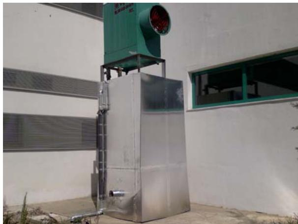
Figure 4.4 Cooling Tower of the Induction Heater Cooling Unit
