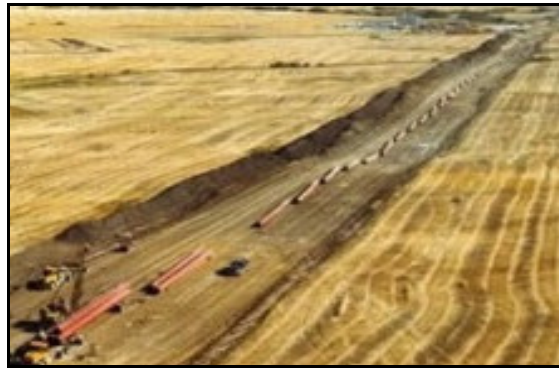
Figure 4.2: Stringing and Bending
