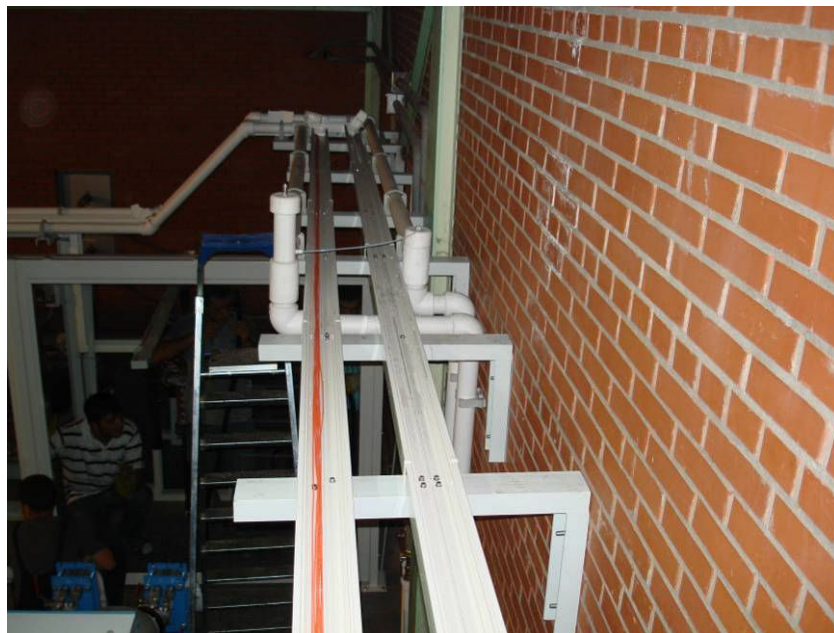
Figure 4.22 Fiber Optic Cable Installation for LTTs
