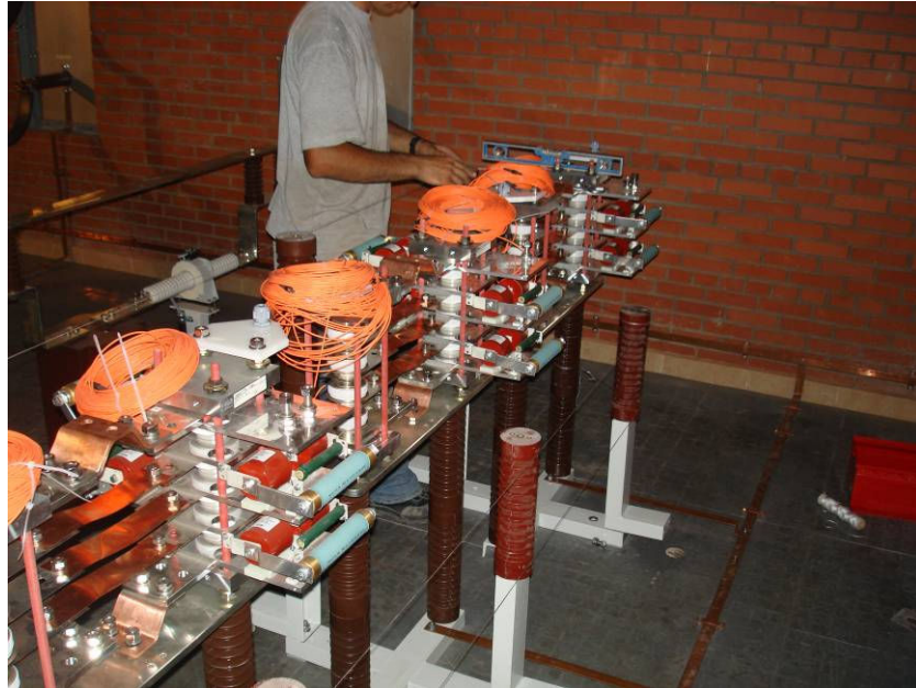
Figure 4.21 Installation of LTT Stacks to Site
