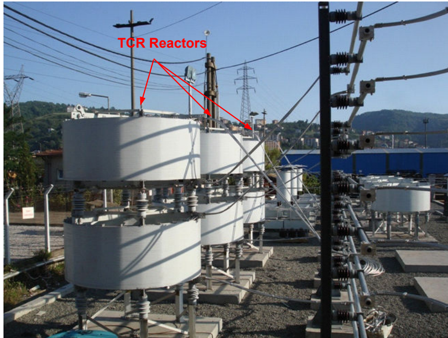
Figure 4.26 Installation of the TCR System
