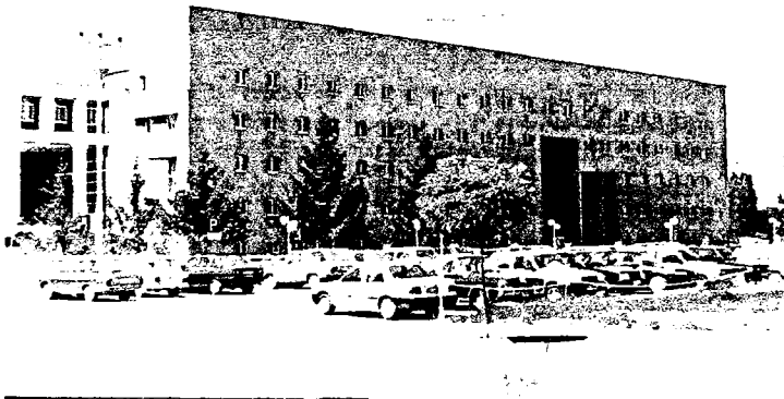
Fig.36.b. Kaysu (Kayseri Water Works), Kayseri, 1980s, Merih Karaaslan; view from the southwest. (Photo by Yusuf Civelek)
