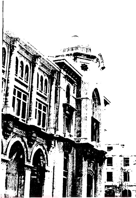
Fig.2.a. Central Post Office, İstanbul, 1909, Vedat (Tek); general view from the northeast. (Photo by Yusuf Civelek)
