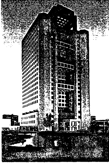
Fig.38.Halkbank Headquarters, Ankara, 1980s, Doğan Tekeli and Sami Sisa; general view. (Mimarlık, 1994, 18)
