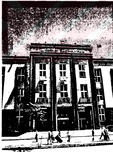
Fig.4.b. Ministry of Health, Ankara, 1926- 1927, Theodor Post and Carl Lörcher; view of the entrance facade. (Photo by Yusuf Civelek)
