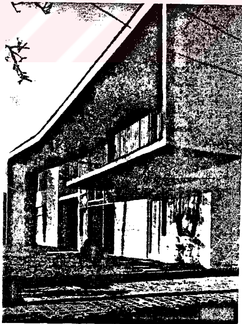
Fig.15.b. House in İstanbul, 1950s, view of the facade. (Kortan, 1971, 82)
