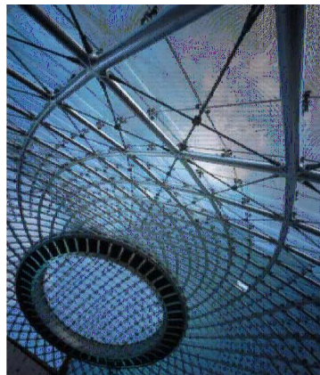
Figure 2.19. Osaka Maritime Museum, the diagrid shell and the ring beam.
