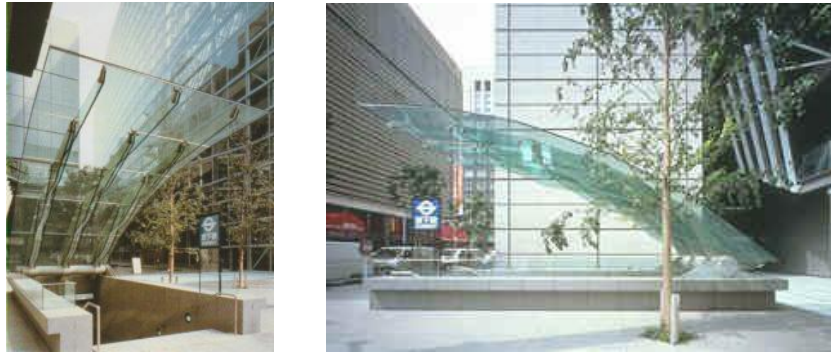
Figure 2.18. Glass Canopy of the Yurakucho Underground Station, Tokyo, 1996.
