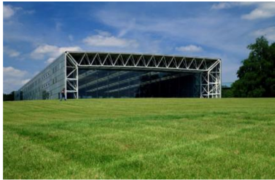
Figure 2.10. Sainsbury Centre for Visual Arts, Norwich, 1978.
