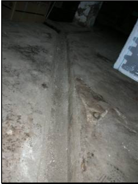
Plate 4.22: Channels providing connection between olive presses and distillation pools, Building # 19.
