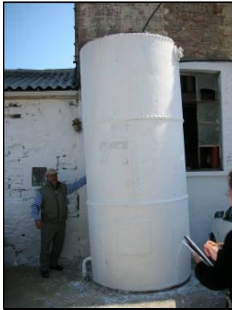
Plate 4.27: Old steam boiler today used as water reservoir, Building #1.
