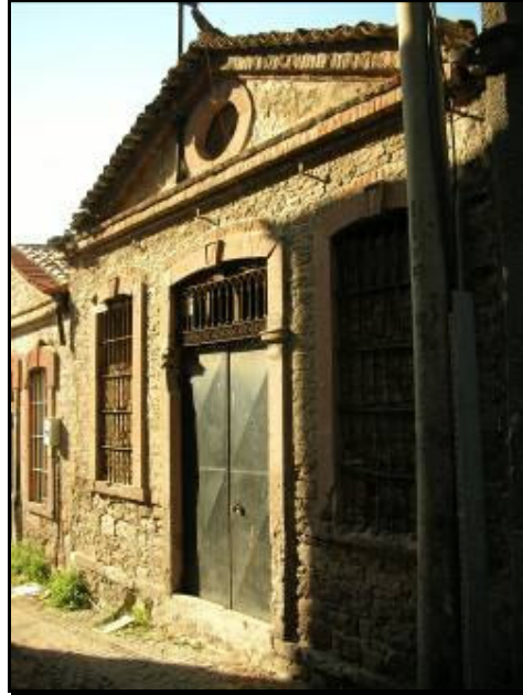
Plate 4.5: 2B type warehouse or workshop, Building # 42.
