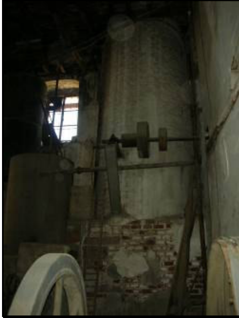
Plate 4.28: Chimney base inside building, Building # 33.
