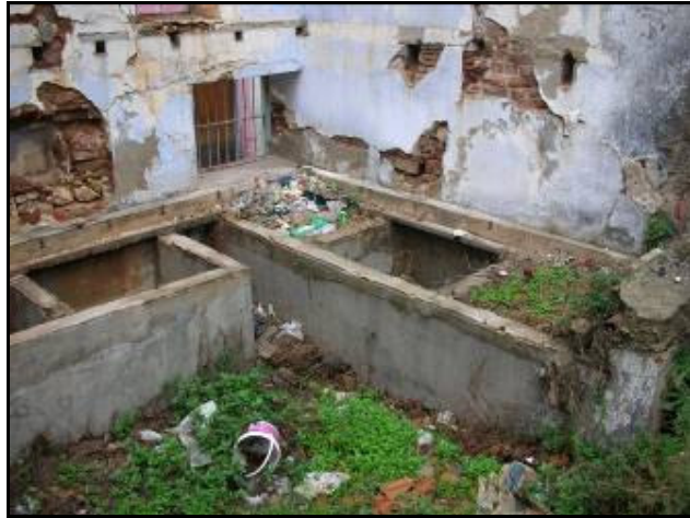
Plate 4.20: Distillation Pools, Building #8.
