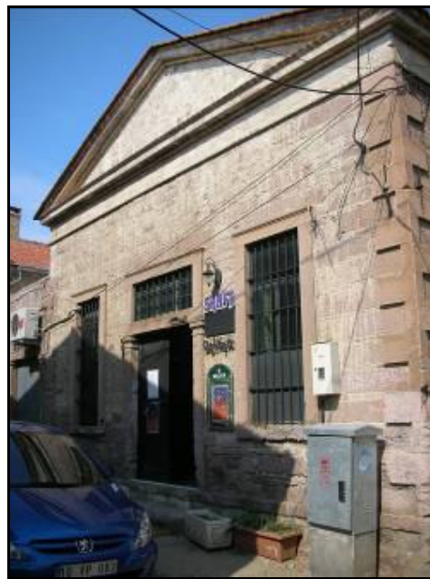
Plate 4.4: 2A type warehouse or workshop, Building # 69.
