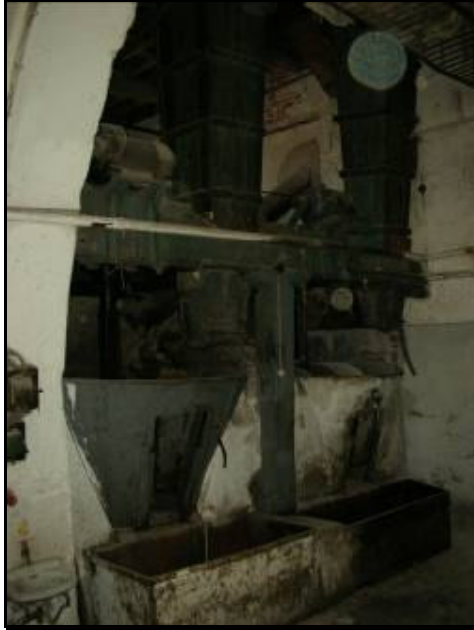
Plate 4.12: Wooden Channels, Building # 33.
