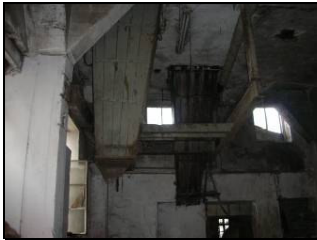
Plate 4.11: Wooden Channels, Building # 1.
