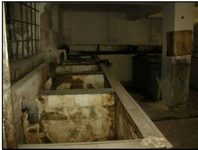
Plate 4.23: Distillation Pools, Building #33.
