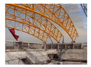
Figure 2.3 Installations of Steel Truss Beams
