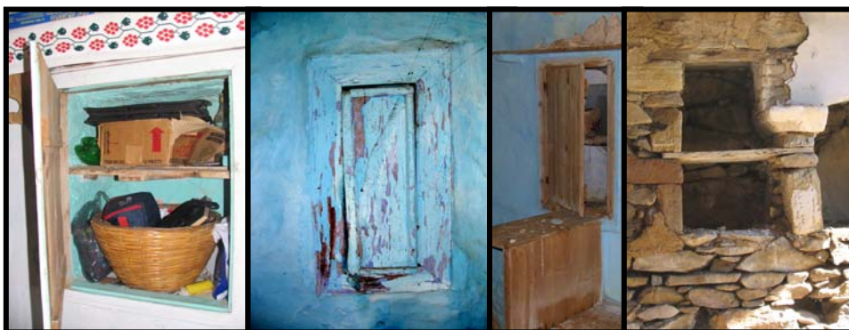
Figure 73 Niches for shelf, either have a lid or not. Sizes cannot be ranged
