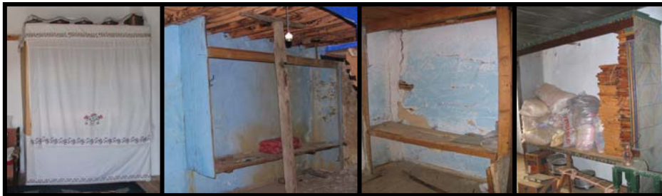
Figure 72 Built in cupboards are either fixed or side to a wall at least from one side
