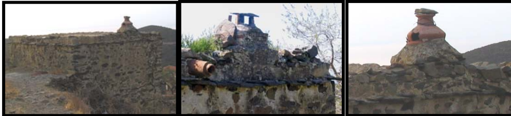
Figure 60 Traditional chimneys are built of stone and topped with baked earth cups
