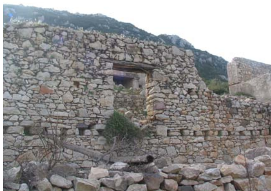
Figure 11 House with white rubble stone from Balıklıova
