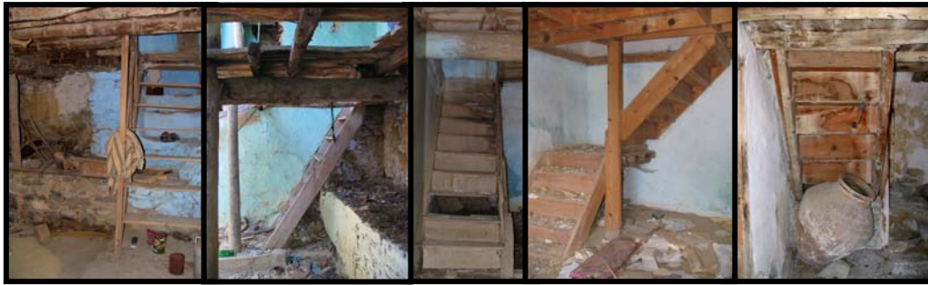
Figure 70 Varieties of timber stairs: straight with or without rise, L shaped and straight with opposite orientation
