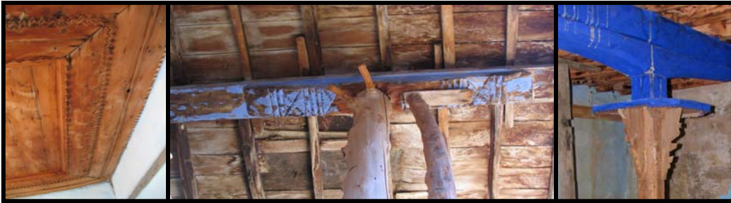
Figure 81 Profiled use of timber elements
