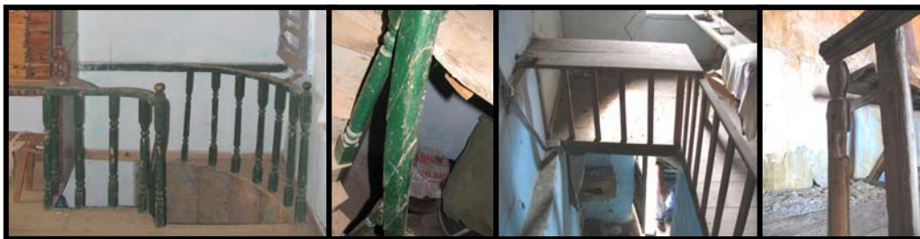
Figure 71 Most stairs are accompanied with simple not profiled balustrade but there are few exceptions which are profiled and painted
