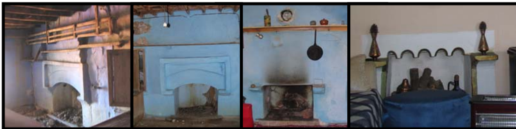
Figure 76 Arched hearth and a timber lath over as a shelf and Flat hearth with tembellik on sides
