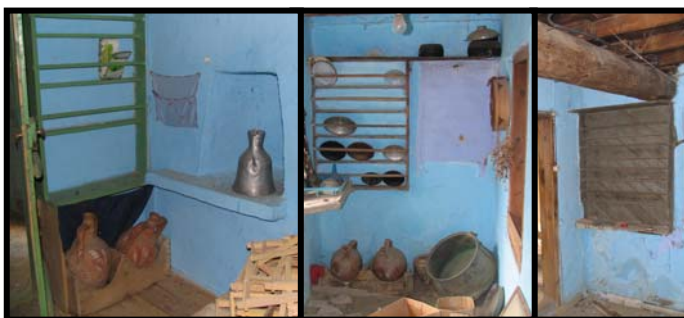
Figure 79 Timber shelves for dishes and boxes for oil and water
