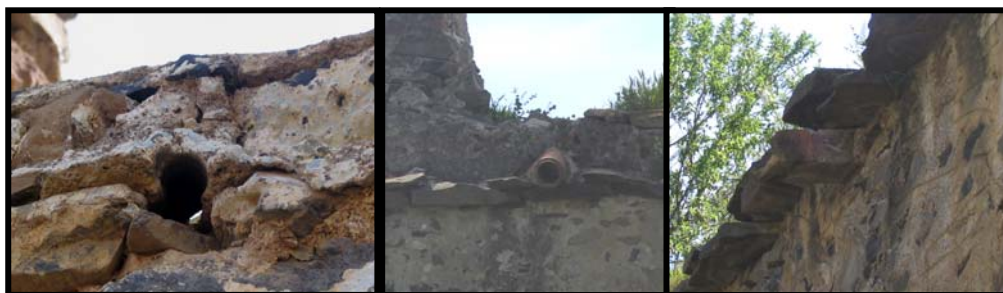
Figure 60 Traditional chimneys are built of stone and topped with baked earth cups
