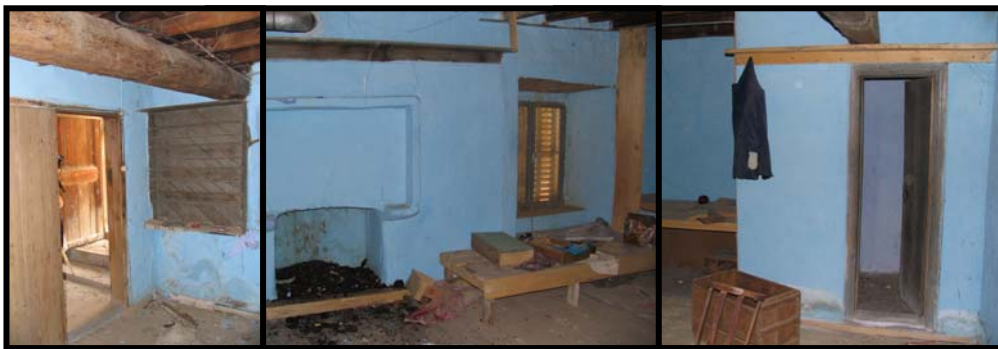
Figure 53 Elevations of the interior walls of ground floor rooms
