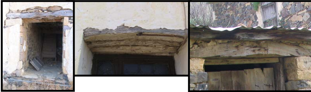
Figure 64 Flat and arched door openings
