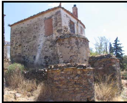
Figure 50 The attached combination of house-stable – circular toilet space. The distinction in the placement of the circular space affects its mass, too. The ones attached to the stable are mostly two storied and the separate ones are single storied.
