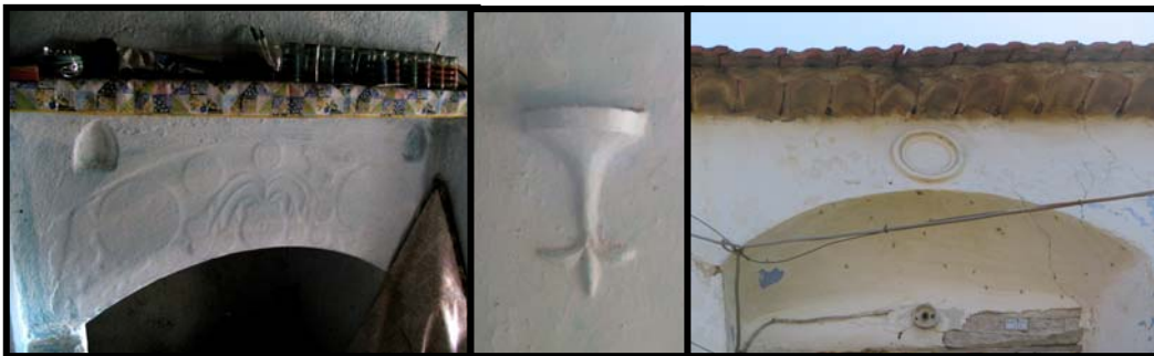
Figure 82 Indoor and outdoor plaster applications
