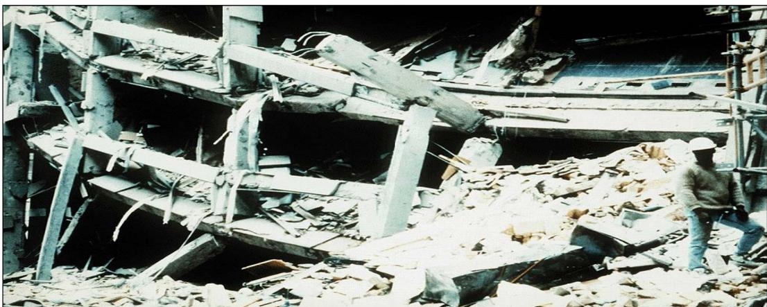
**Figure 1:** Post-Incident View of Building Damage from the 1992 St. Mary's Axe Bombing Incident in London. (From work of Krauthammer, 2003)
