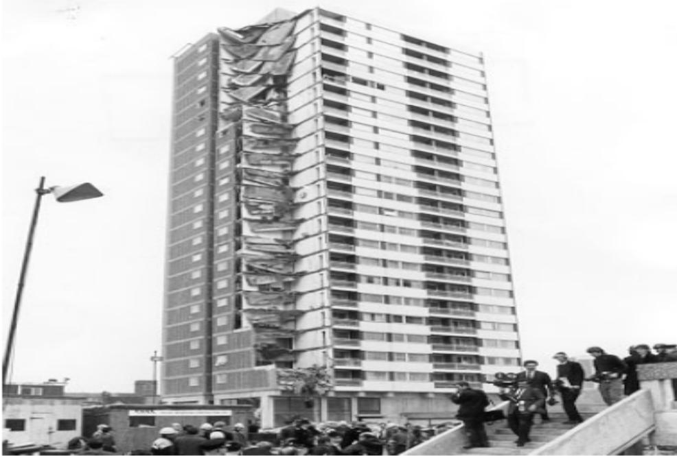
**Figure 16:** Ronan Point building after 16 May 1968 collapse.
