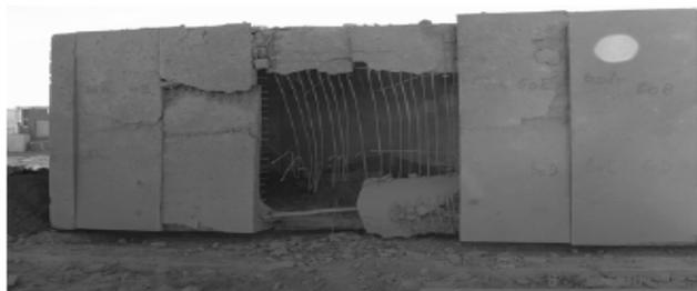
**Figure 13:** Breaching failure due to a close-in explosion of 6000kg TNT equivalent.
