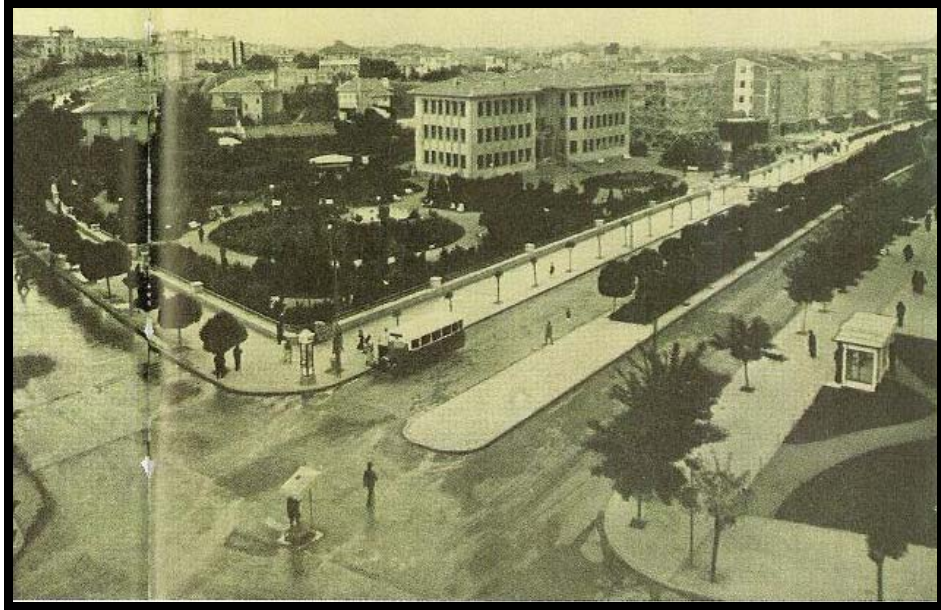
Fig. 17. Kızılay Square, Kızılay Building with its garden, 1938 Source: Çankaya , 1991: 97
