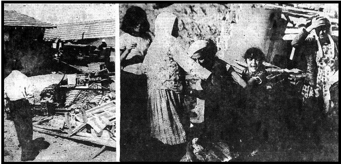
Fig. 40. Destruction of squatters, July 1968
