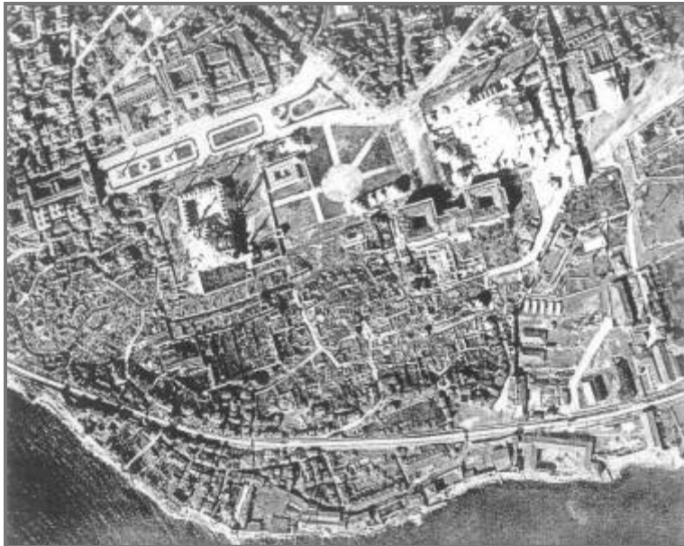
Figure 3.28: View of land of Grand Palace in 1918. The trace of 1912 fire is seen SOURCE: Müller-Wiener, p.230
