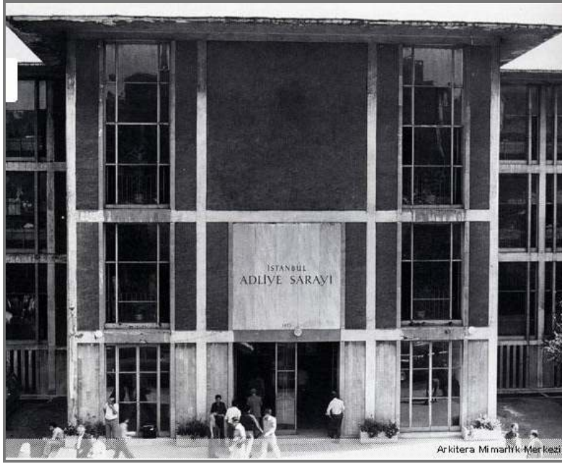
Figure 4.9: The built part of Law Court in Sultanahmet SOURCE: ⇒WWW, Internet], Address: http://www.arkiv.arkitera.com [Accessed: 09.12.2007]
