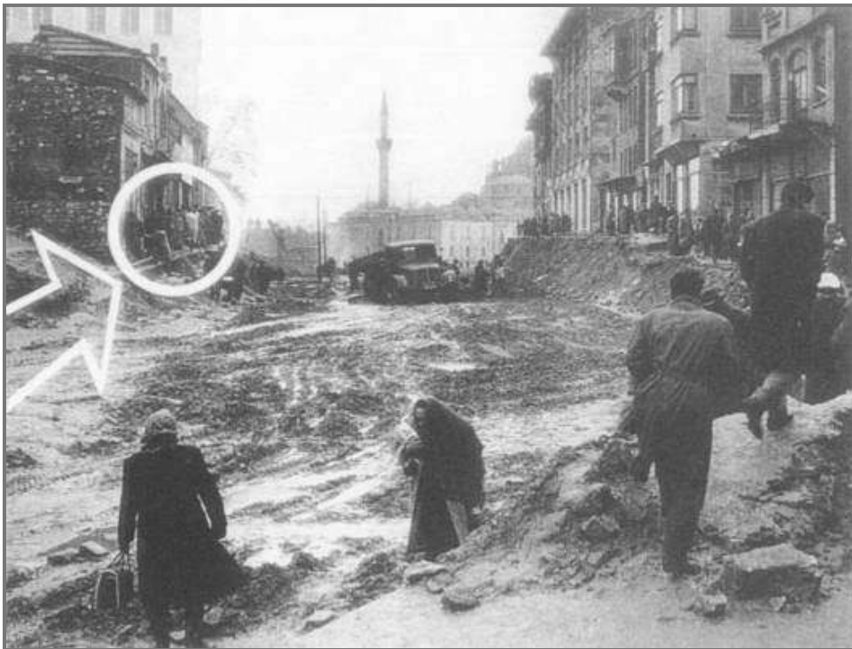
Figure 4.20: Expropriation on Vezneciler Street connecting to Beyazıt Square. SOURCE: Tanyeli, “Türkiye’de Metropol Kavrayışı”, p.94
