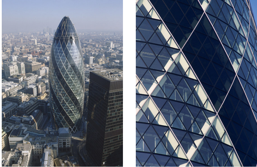
Figure 2.3 Triangulated façade of 30 St Mary Axe. 33
