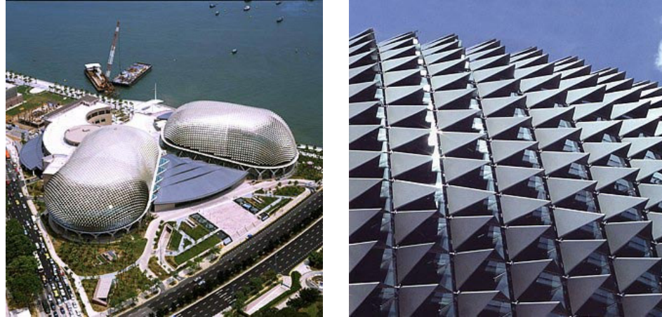
Figure 2.2 The complex roof form of Singapore Art Centre 16 .
