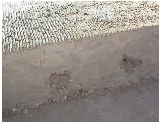
Figure 1.10 Plastic shrinkage because of bleeding *
