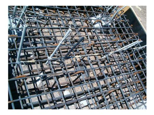
Figure 3.2 Installation of the earth pressure cell beneath the raft
