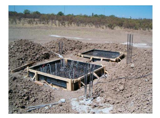
Figure 3.3 Construction of model piled raft
