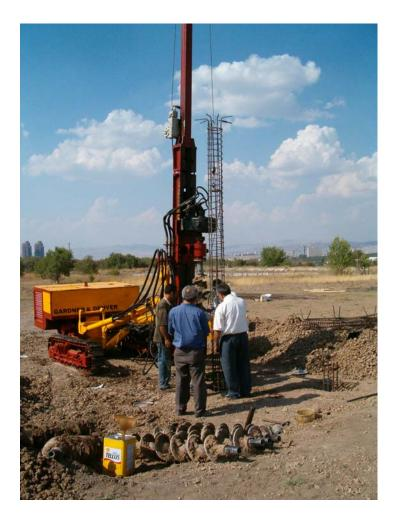
Figure 3.1 Construction of bored piles
