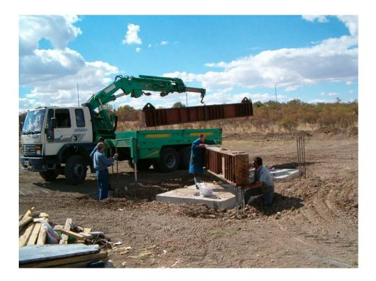
Figure 3.4 Replacement of steel reaction beams
